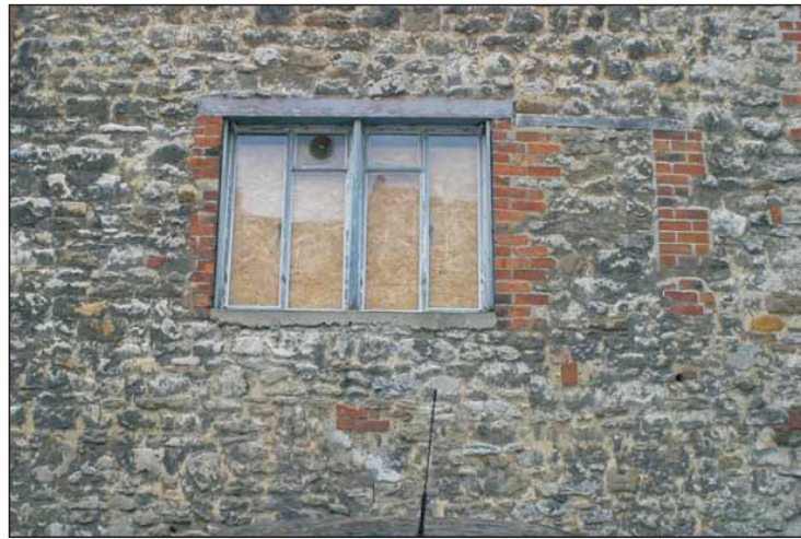
Plate 1. Rear of No. 28 St Michael's Street showing the two different window phases (wall A)
