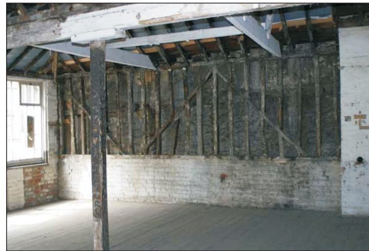
Plate 7. The west wall of St Michael's Street showing the frame for boarding and the wall of No. 34 built of timber with stone and mortar infill. Two windows have been blocked (wall C)
