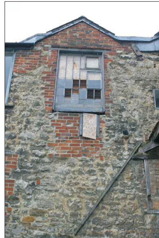
Plate 5. Insertion of window and building at the rear of No. 30 St Michael's Street (wall A)
