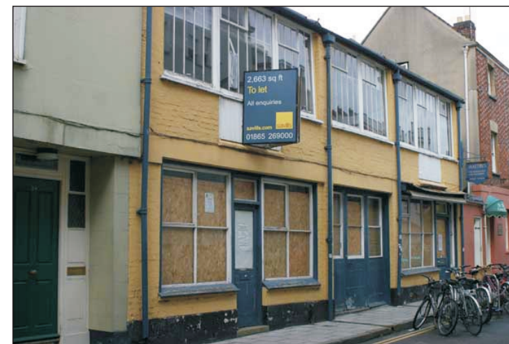
Plate 10. General view of No's. 28-32 St Michaels Street. The front of the building may have been replaced wholly or partially (Phase 7), (wall F)
