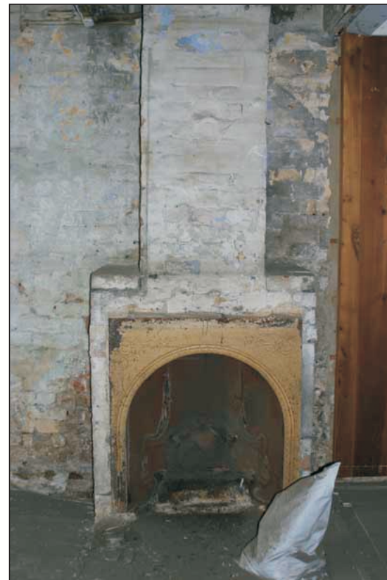
Plate 9. The mid - late 19th Century fire place and chimney breast butting up against the existing east wall (wall E)
