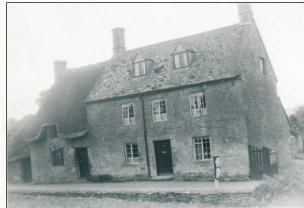
Figure 5. Historic photograph of 28 Crockwell St showing side-building and access on left hand side
