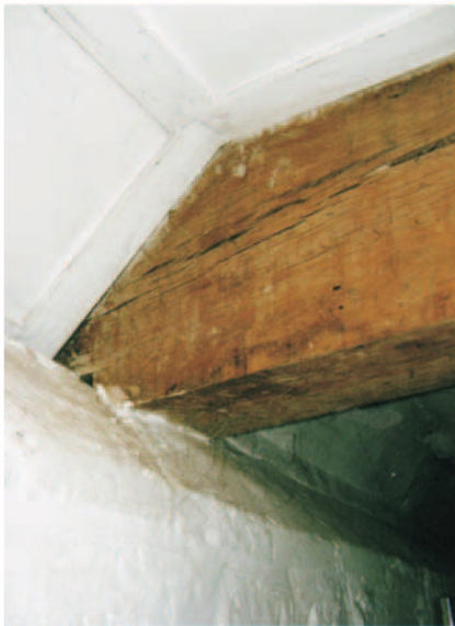
35. End of tie beam resting on west wall
