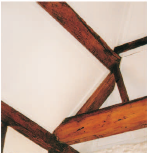
39. Pole and plate purlin. South east corner.
