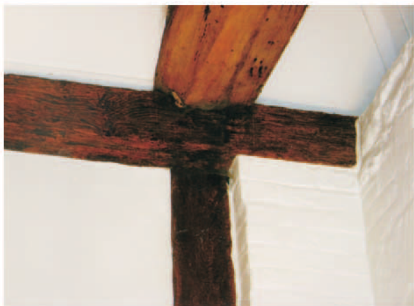
37. Pole plate and tie beam. South east corner.
