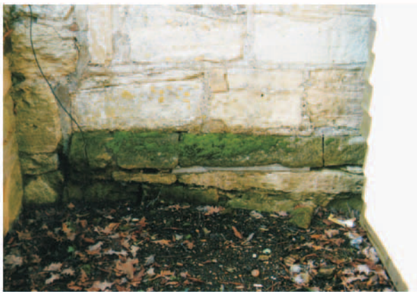
16. Water table to "garden wall" to the south east side.
