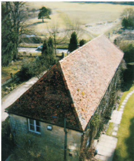
7. View of annexe from top of tower
