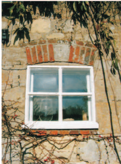
11. South window. Note stone keystone
