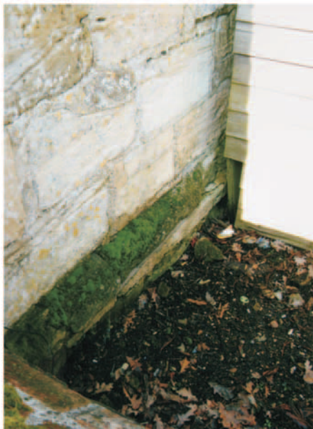
15. Water table at foot of garden wall indicating continuance of building.
