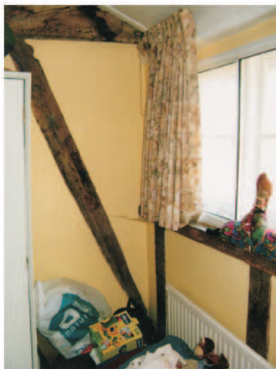
40. Strut in bay 2 from north. First floor.
