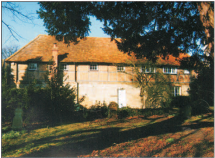
1. East Front. Note Timber framed and brick nogged upper storey. Also hipped tiled roof.
