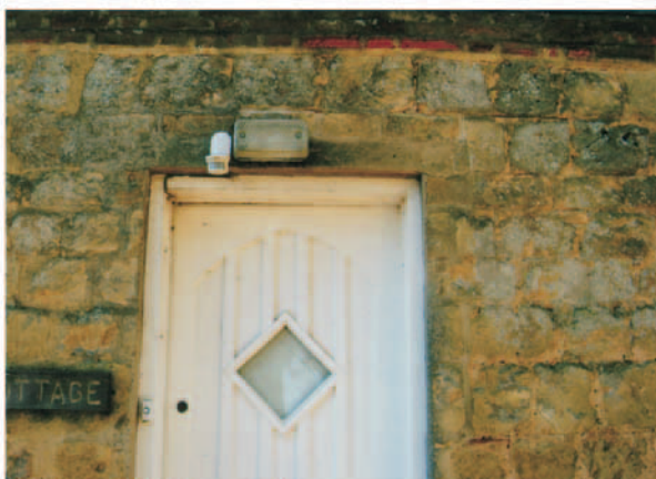
24. Concrete lintel over east door
