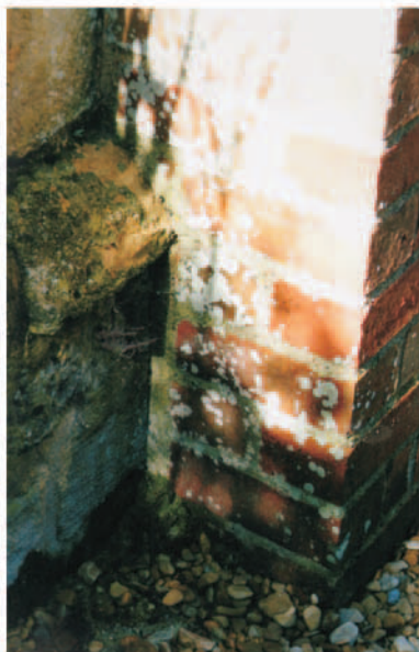
23. Detail of water table and 1950s chimney
