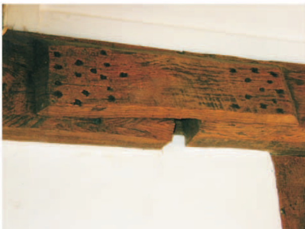
38. Oak plate nailed to pole plate east side above stairs
