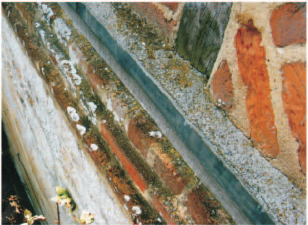
18. External view showing central position of cill plate
