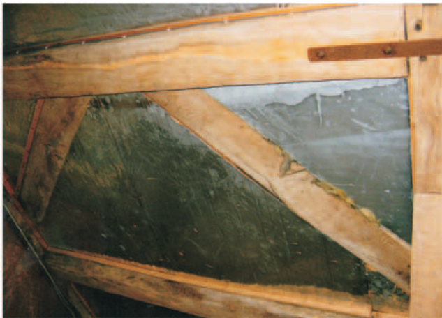
36. Windbraces in place between upper and lower purlins. West roof
