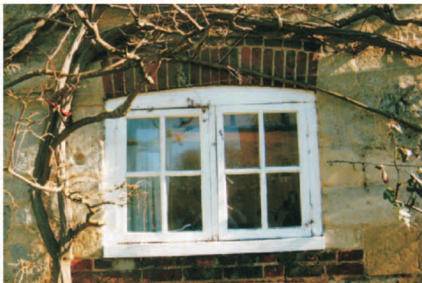
12. Window in west front
