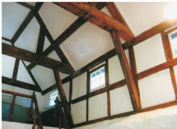
28. East wall looking north east. Note supports nailed to tie beams
