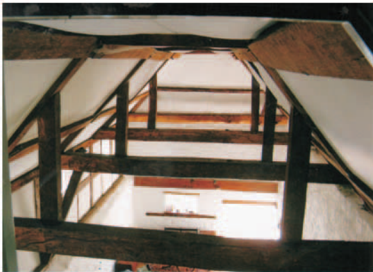
26. View of roof from balcony. Note two ranges of purlins.
