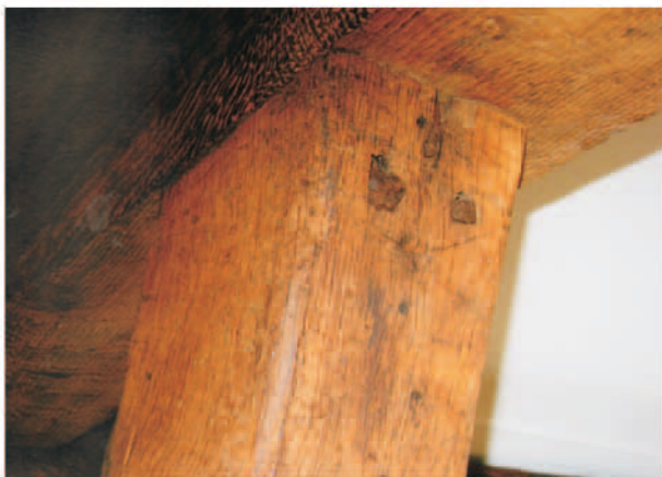
33. Strut above stairs nailed into position.
