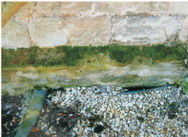
19. Water table. East wall.
