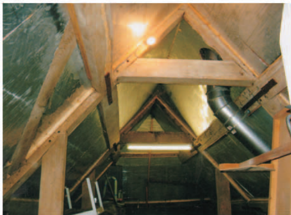
30. Apex of roof looking north. Note high position of collars
