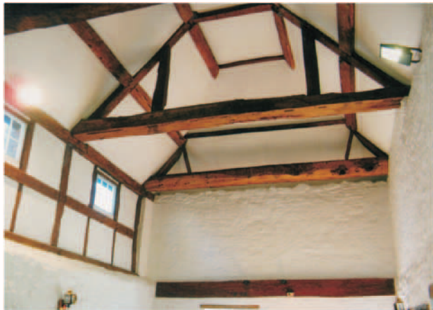
29. East wall looking south east.
