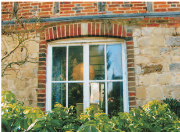
9. Window. North end, east wall.
