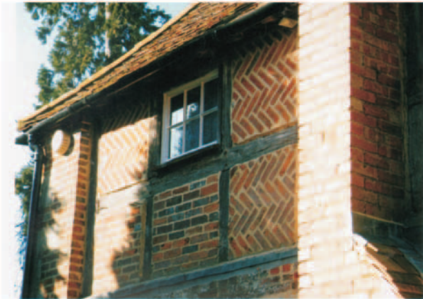
3. East wall at south end. Note herringbone panels of brick work
