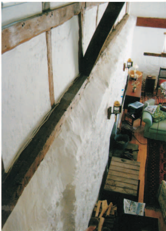
43. View showing central position of cill plate on masonry east wall.
