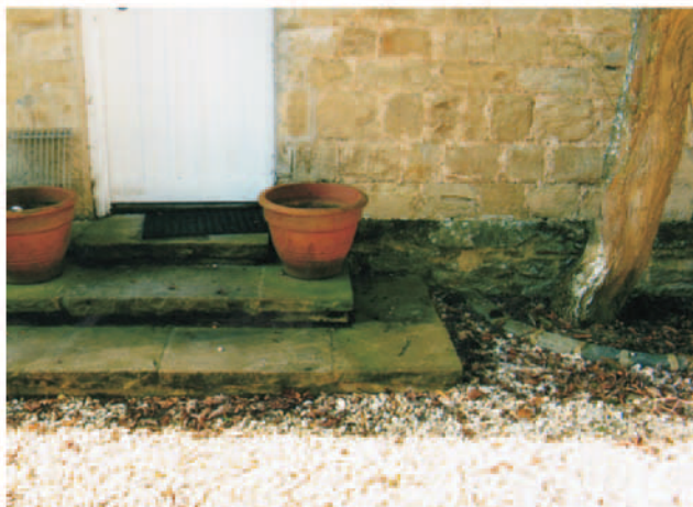
20. Steps up to east door. Note water table.
