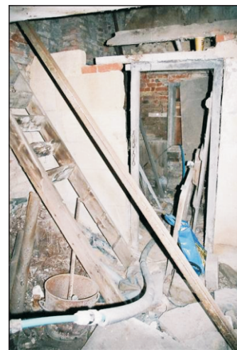
Photograph taken during assessment showing ladder to first floor
