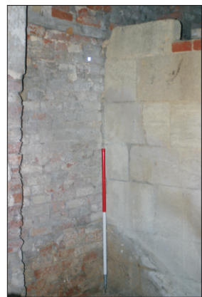
West elevation and stone wall in passage
