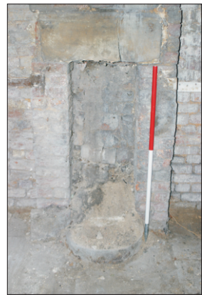
Fireplace in west internal elevation
