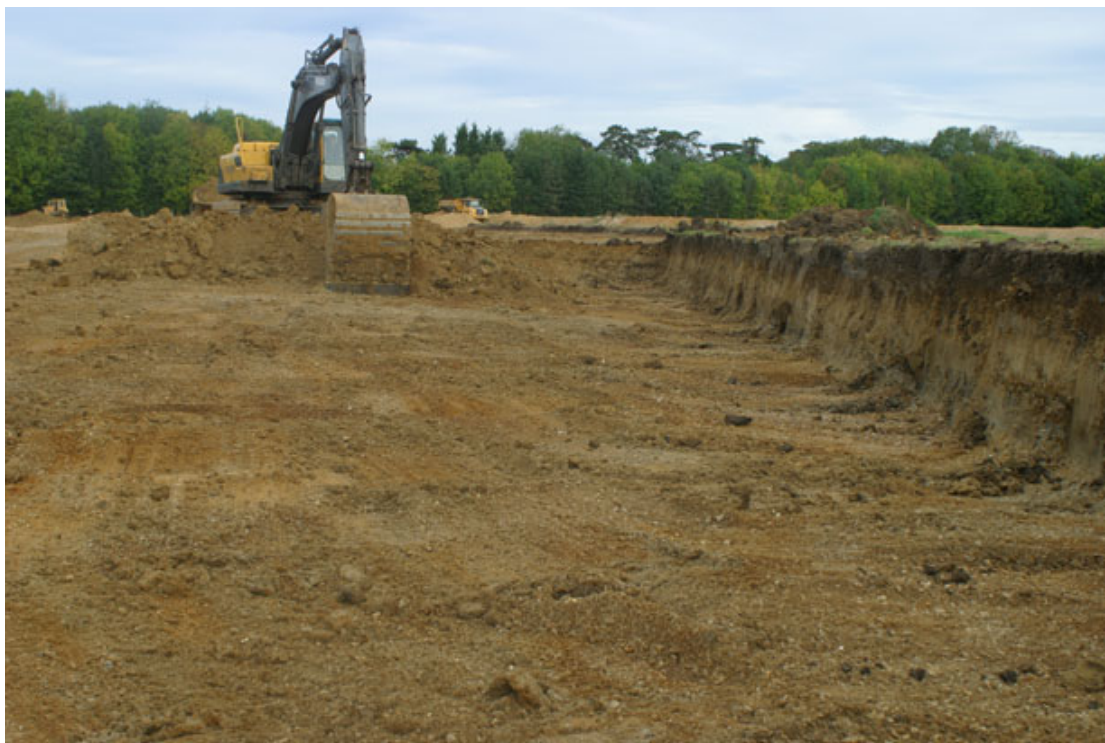
Plate 1. Removal of alluvial clay in progress in October 2011
