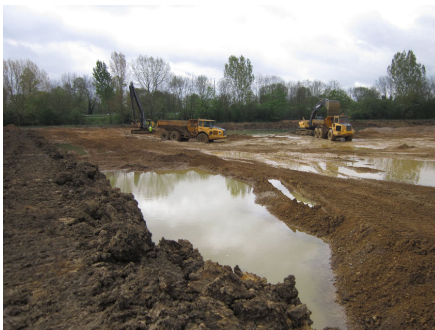
Plate 7. Work during poor weather in May 2012
