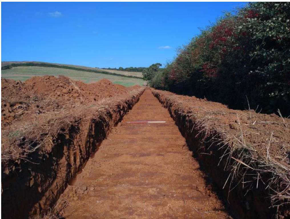
Plate 23: Area E2 – Topsoil stripping post-excavation, camera facing north-east
