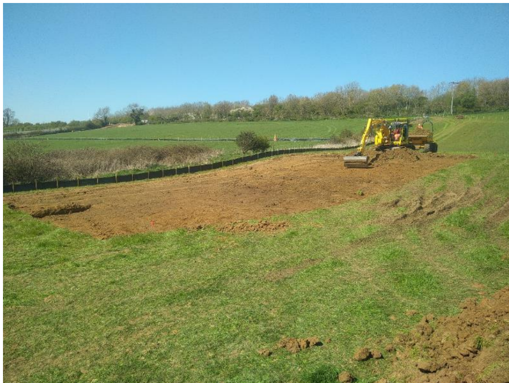
Plate 1: Area C1 – Topsoil stripping, camera facing north-west
