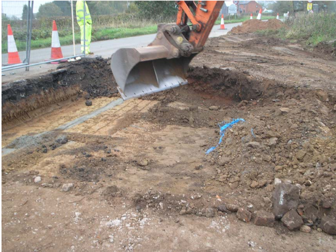
Plate 3 Working shot of topsoil stripping looking W
