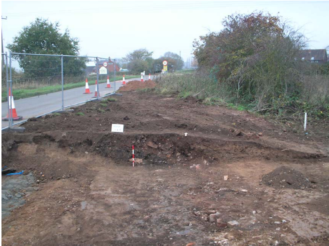
Plate 7 Ditch 107 looking N
