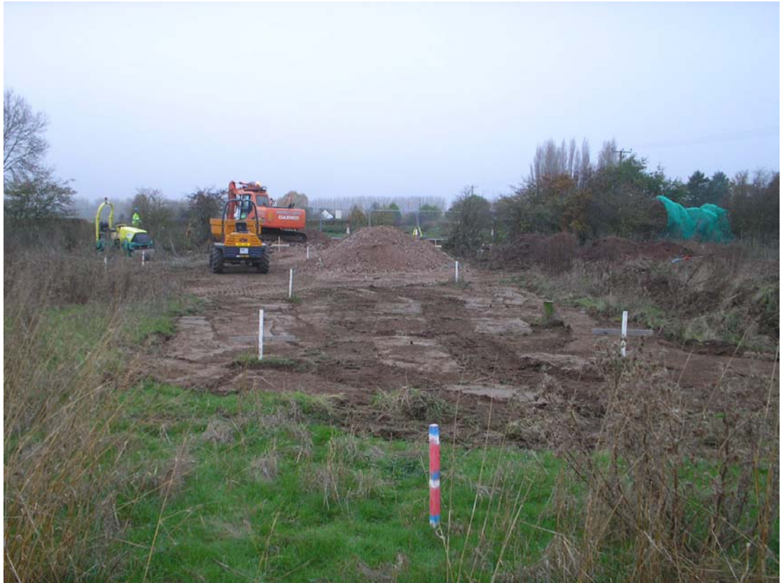
Plate 5 Working shot of site clearance looking W
