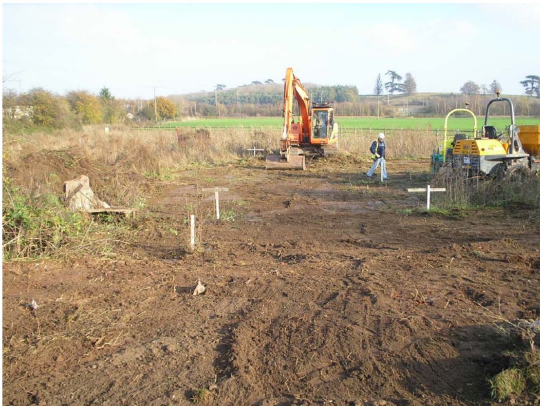
Plate 4 Working shot of site clearance looking NE
