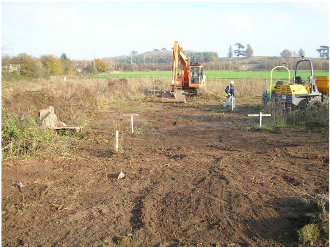
Plate 2 Machine clearing site looking NE
