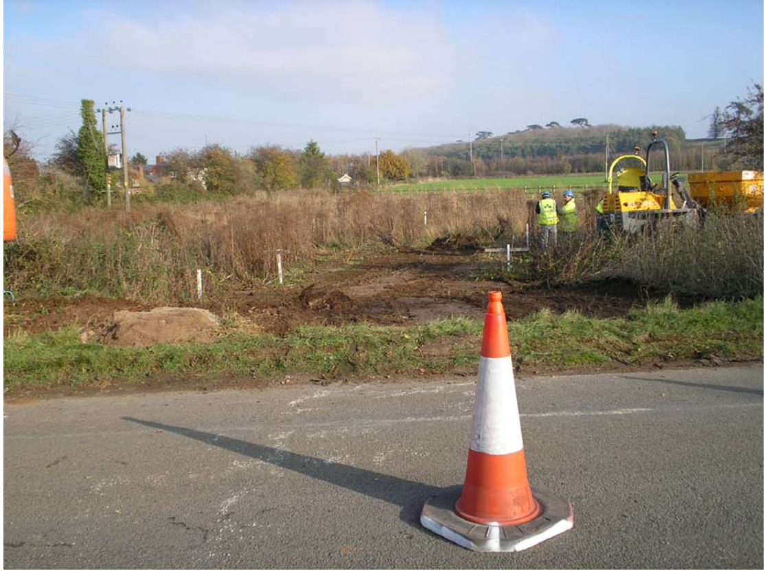
Plate 1 Site clearance for access track looking NE
