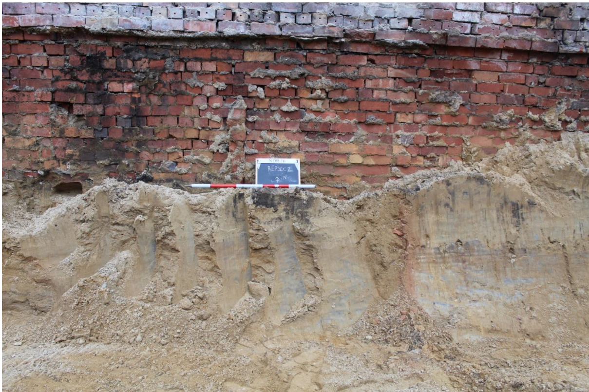
Plate 2. View of site section. Facing north-northwest.
