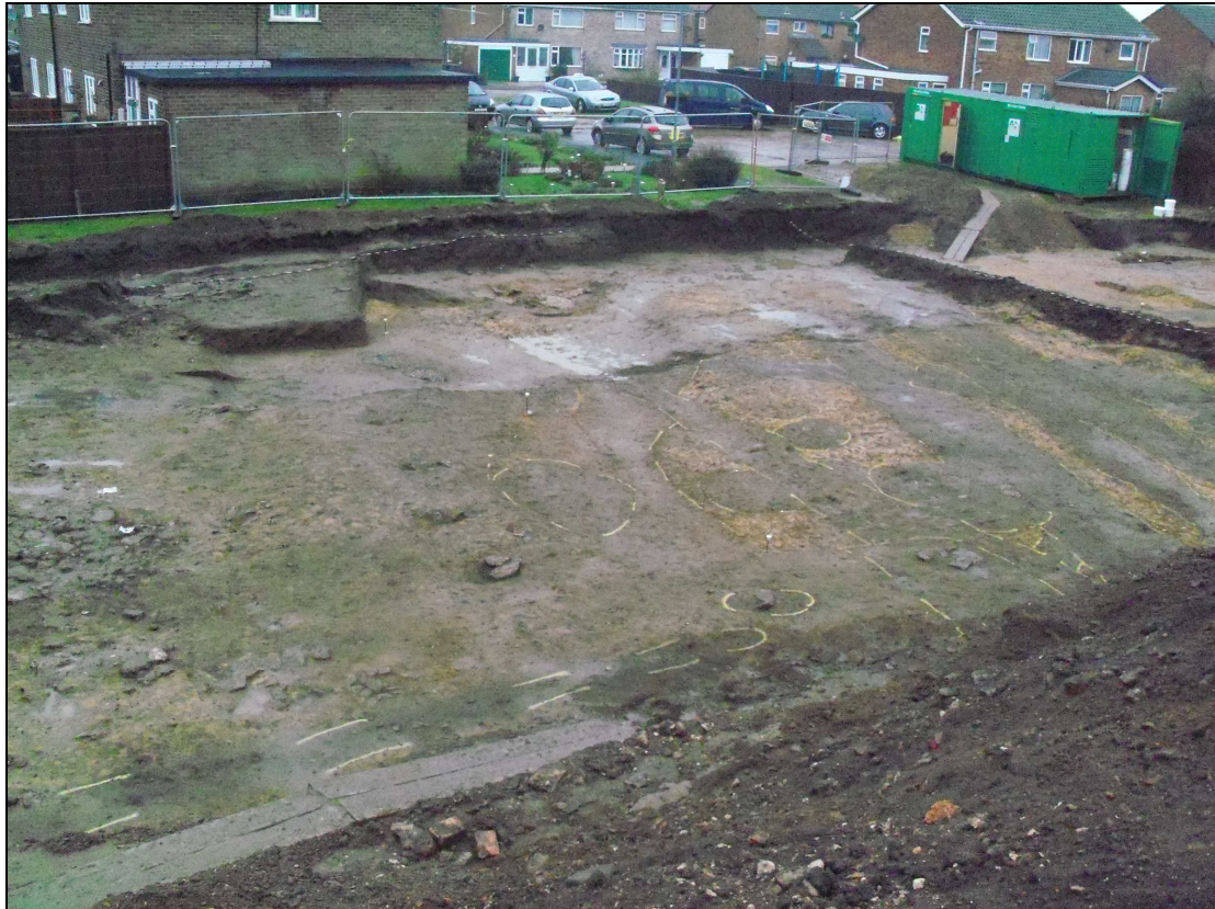
Plate 3: Northern part of site following cleaning
