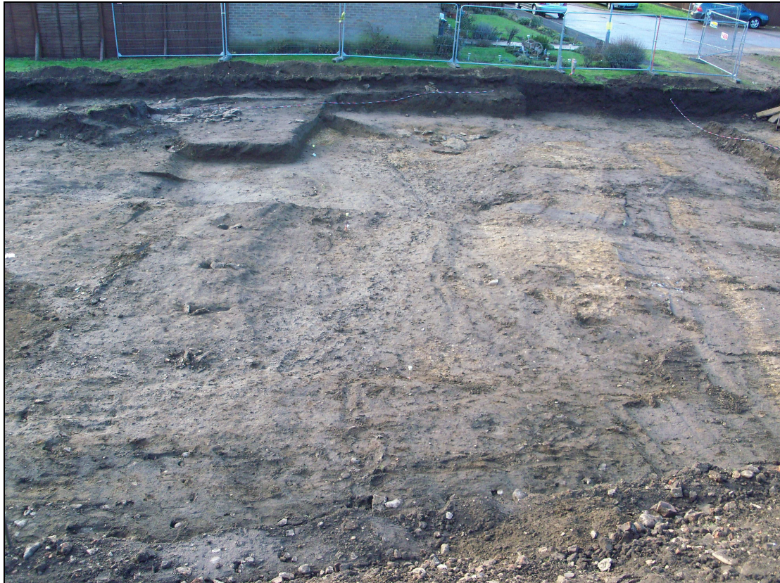
Plate 1: Initial strip of site, looking west
