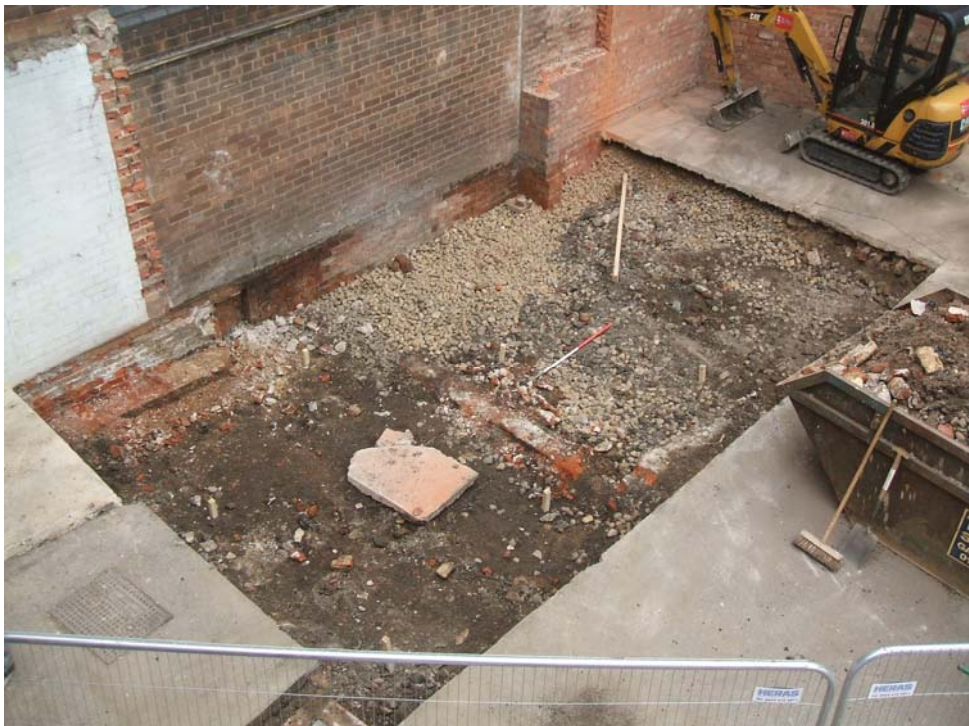
Plate 2: The development area following machine clearance of overburden
