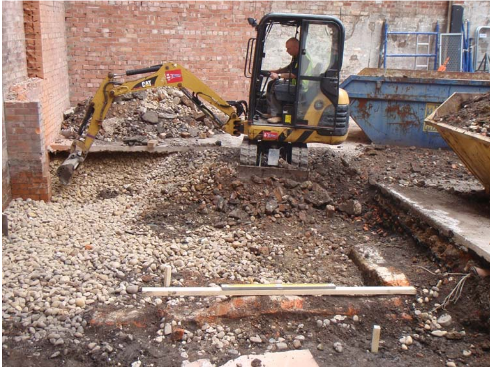
Plate 1: Machining off overburden from the development area
