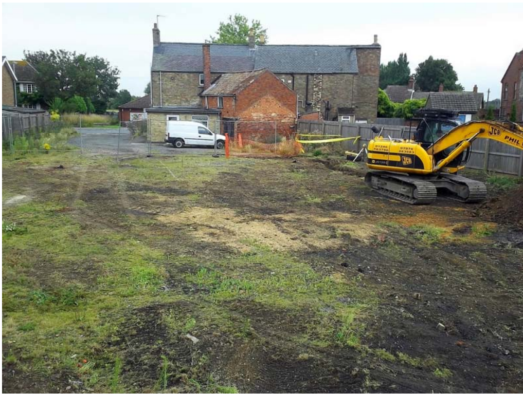
Plate 1: pre-excavation site shot, camera facing north
