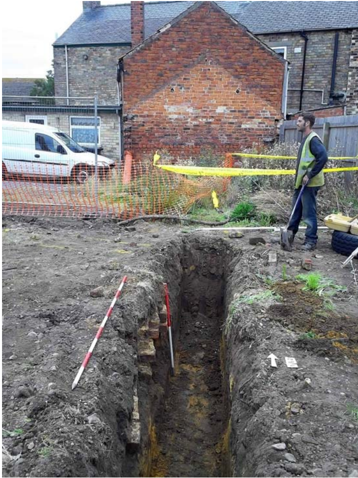
Plate 3: Wall 102, showing alignment with wall scar on standing building
