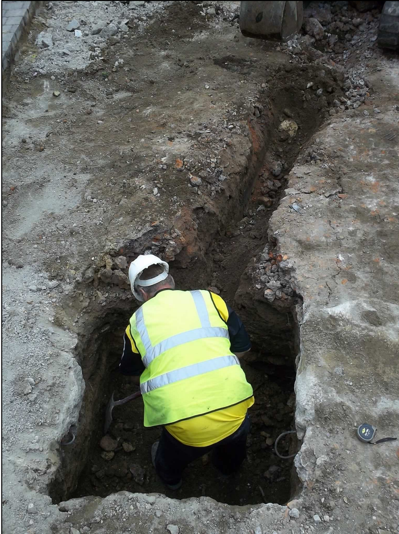
Plate 1: Excavation of Pit 1 and connecting trench.
