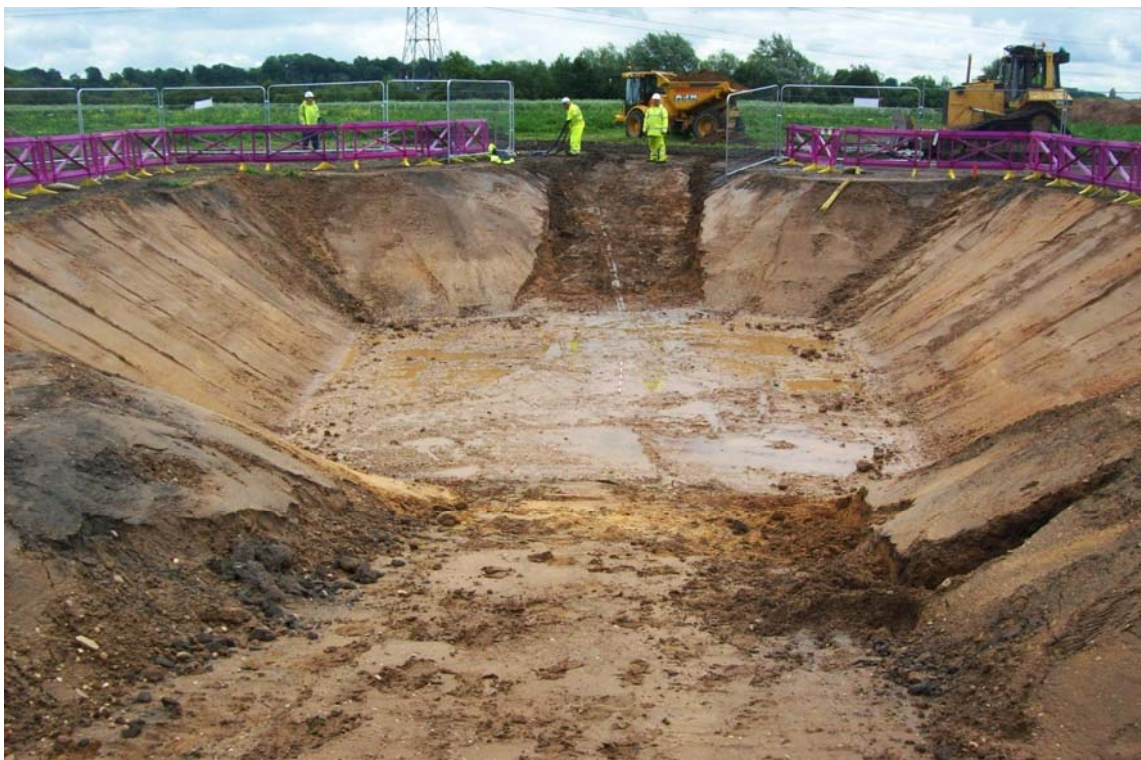
Plate 9: Area G following excavation
