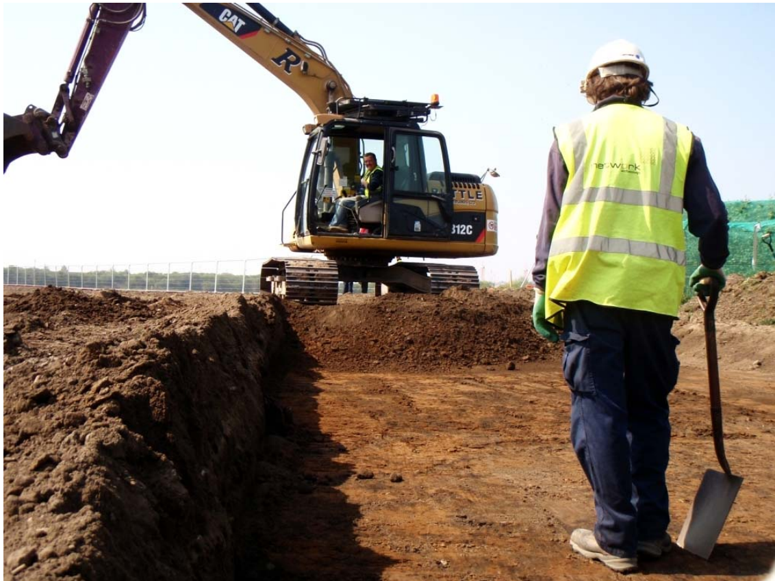
Plate 3: Working shot: Chris Casswell monitoring topsoiling in Area A
