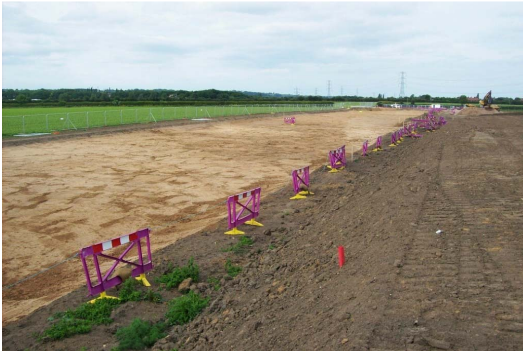
Plate 2: Area A following topsoiling/subsoiling, camera facing north
