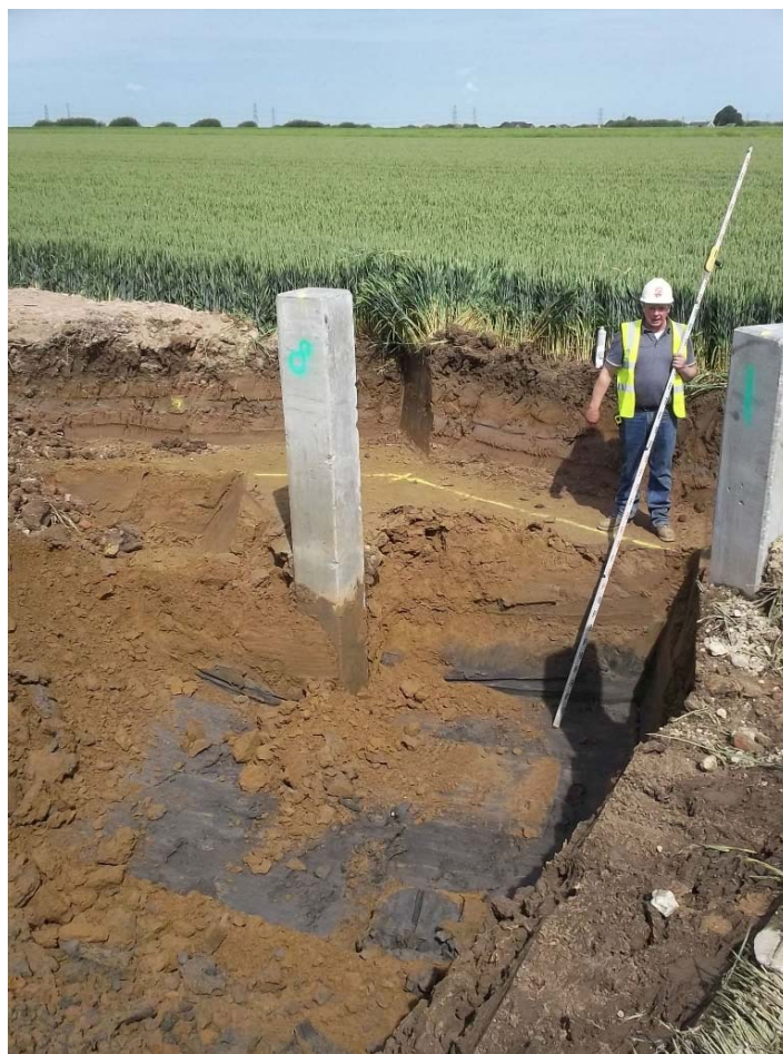
Plate 2: Excavation in progress: top of peaty silt exposed below c.2m of overburden
