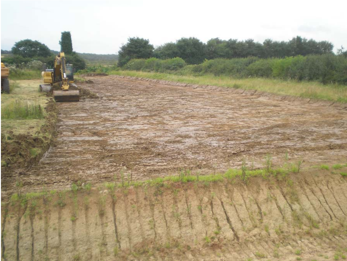
Plate 1: Working shot of New Best Red Quarry topsoil stripping, looking south-west
