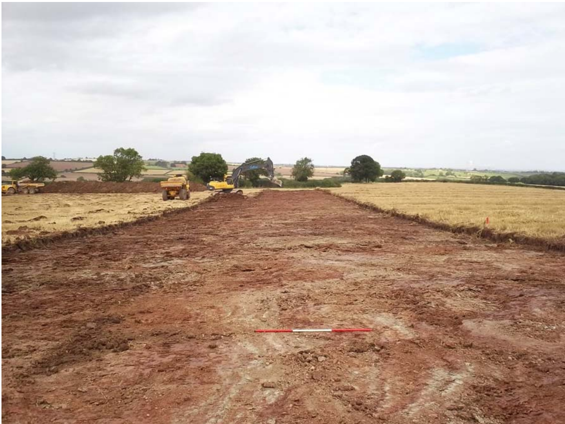
Plate 2: Working shot of Cream Quarry topsoil stripping, looking north-east
