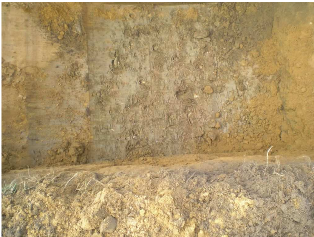
Plate 3: Natural ironstone deposits exposed in base of cable trench
