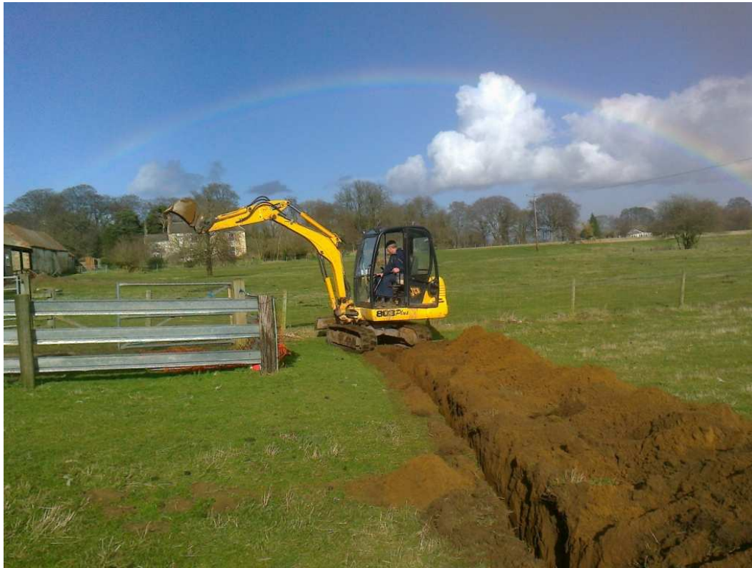
Plate 2: Looking north along cable trench towards Holme Hall
