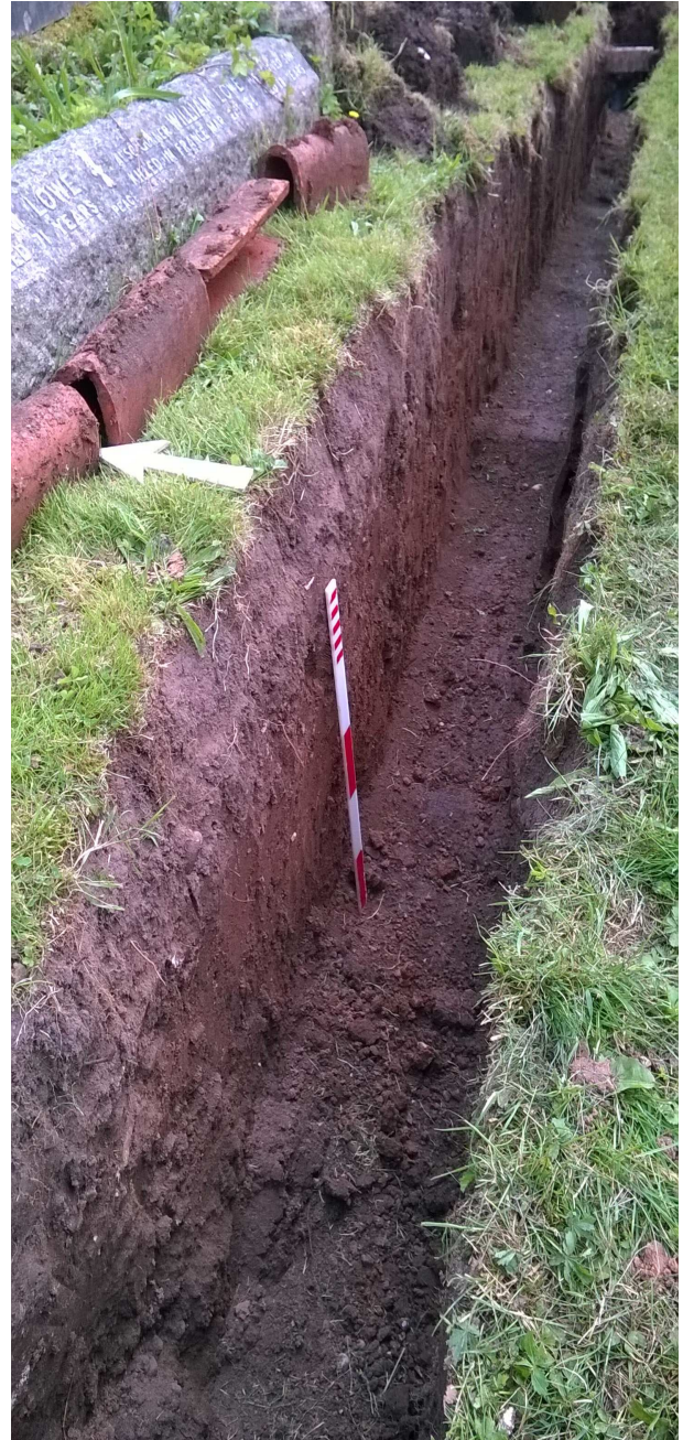
Figure 9: South trench, fully excavated, the south side of base disrupted by drain (130), scale 0.5m
