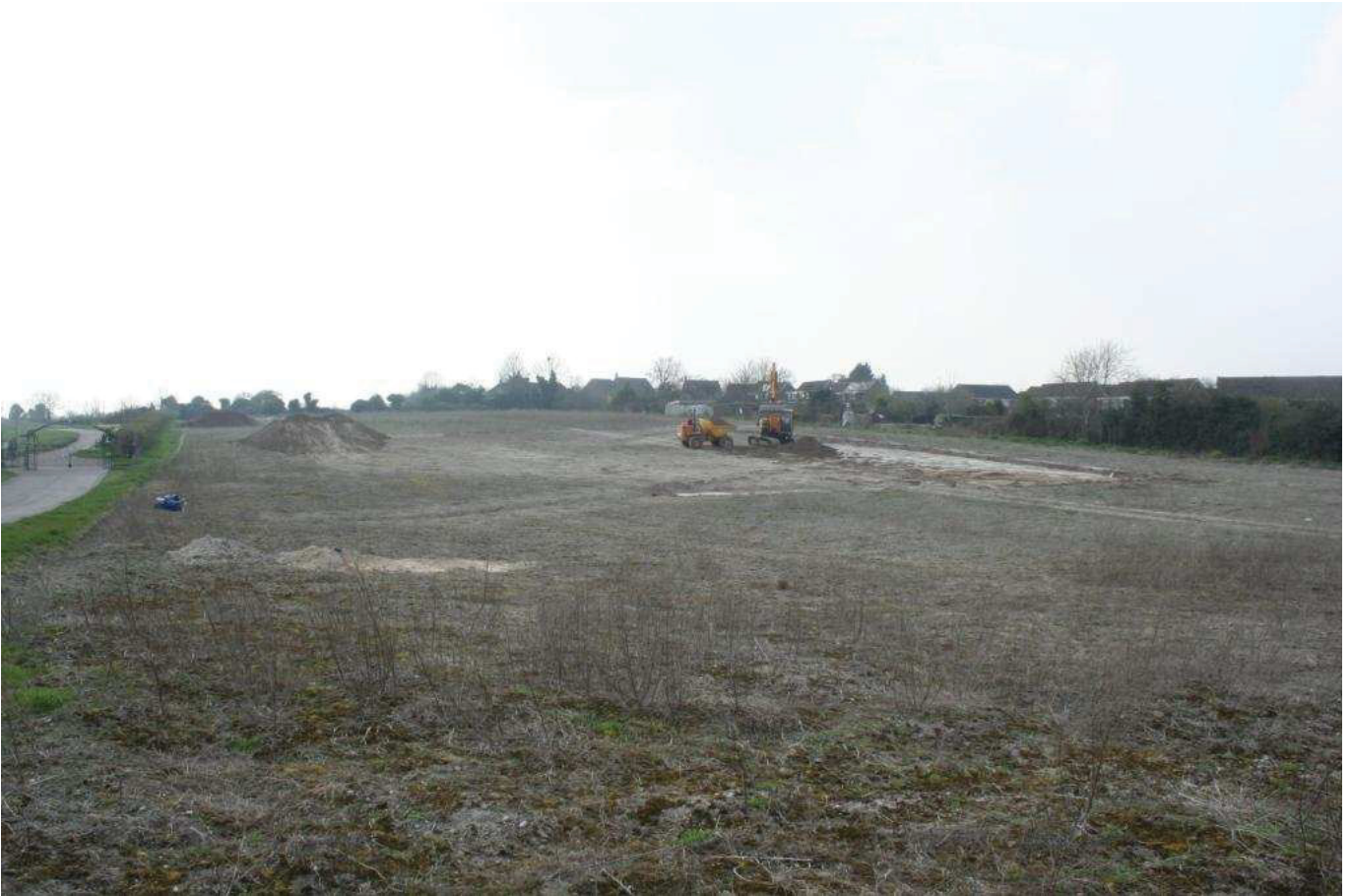
Plate 1: General view of the development area during stripping. Camera facing northwest
