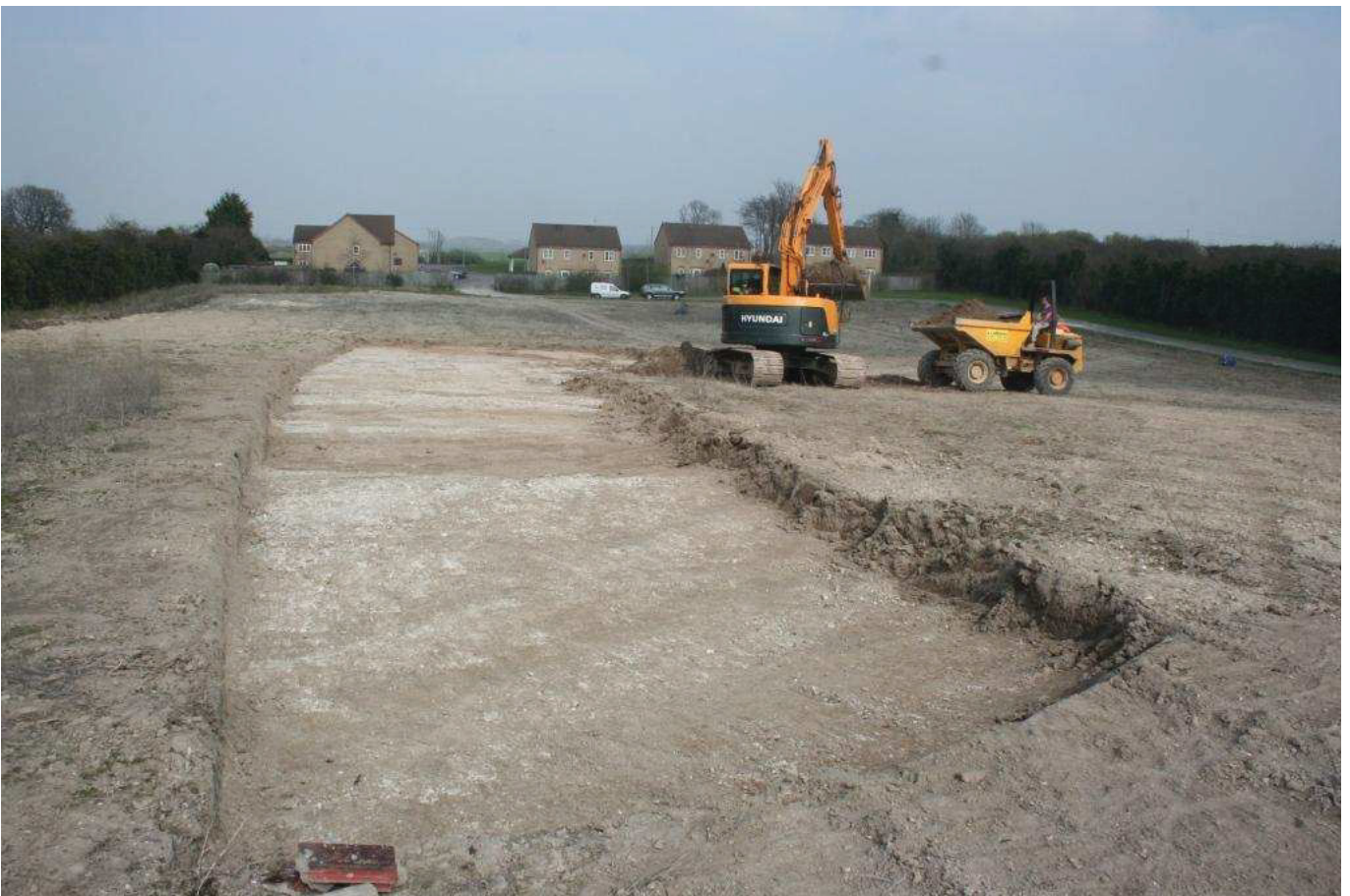
Plate 2: General view of area 2 during stripping. Camera facing northeast
