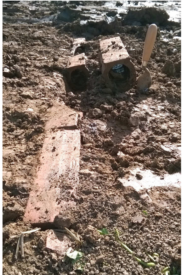
Figure 12: Distinctive flat-topped ceramic drain, western end of track to Flixborough Wharf, looking south
