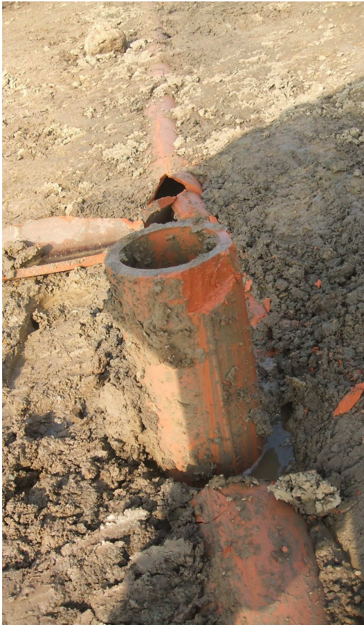
Figure 11: Ceramic land drain in WT5, looking west
