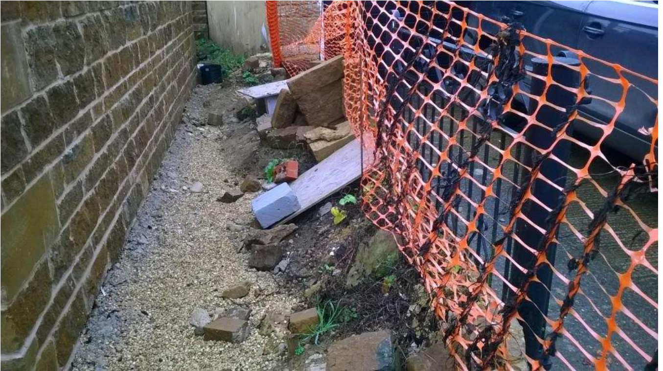
Plate 10: Location of trench 2 pre-excitation. Camera facing east
