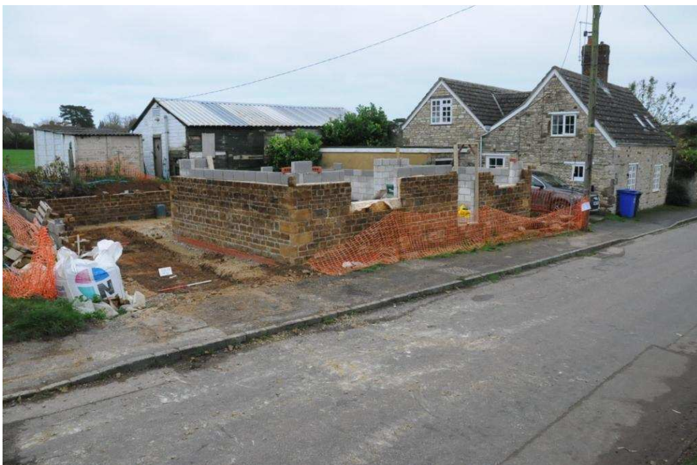
Plate 2: General view of the PDA. Camera facing southeast
