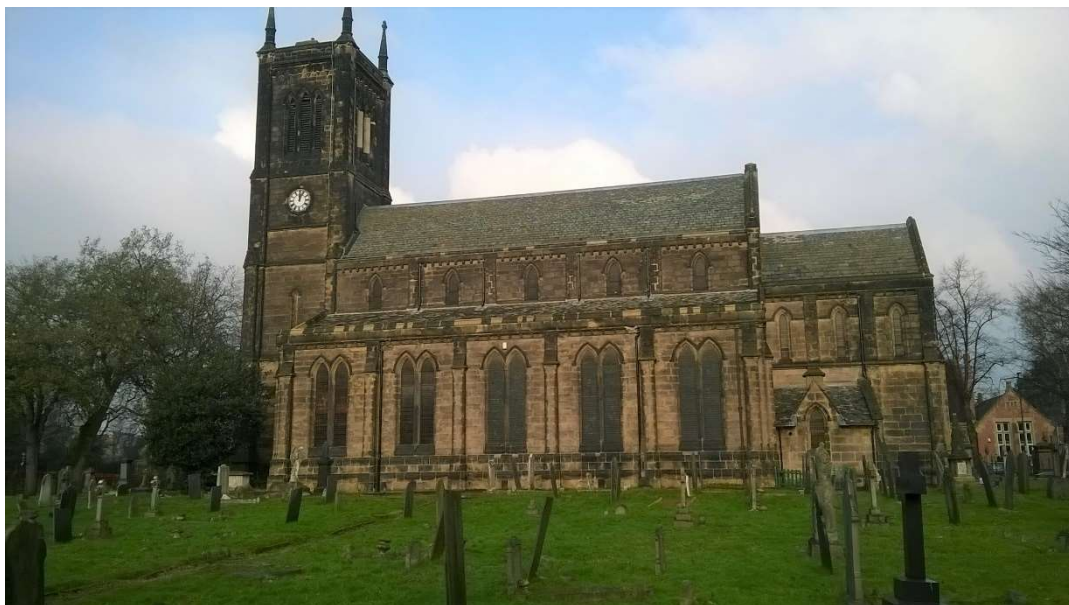
11: View of the church from the south part of the churchyard showing the arrangement of gravestones in rows, with gaps where memorials have been lost
