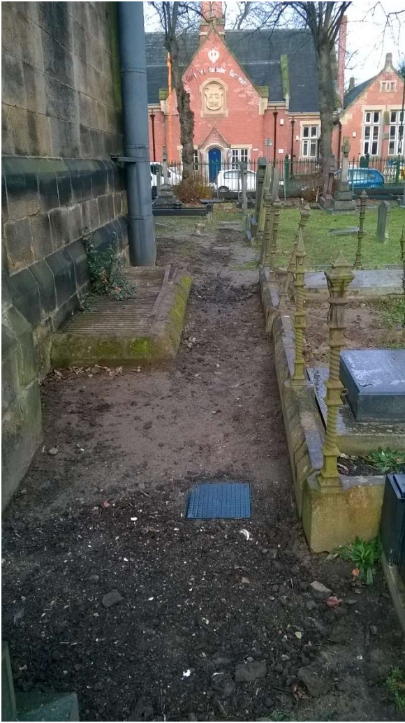
9: View northward along the east end of the chancel, showing the infilled drainage trench between the boiler room vent and the kerbed graves
