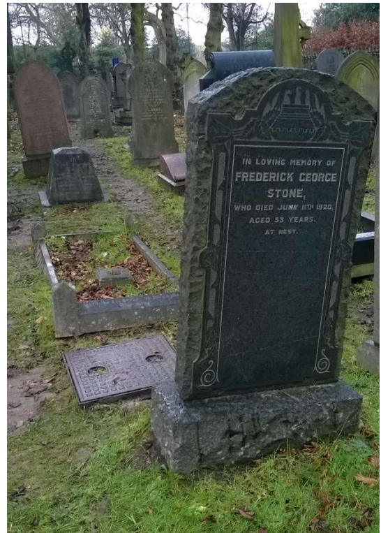
7: The existing manhole between the eastern end of the church and Church Street
