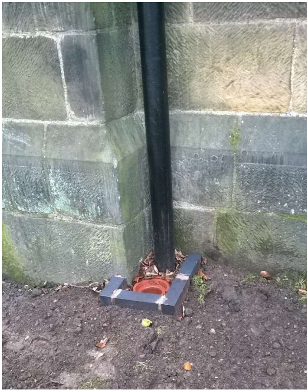
6: Newly constructed gully against the north wall of the chancel
