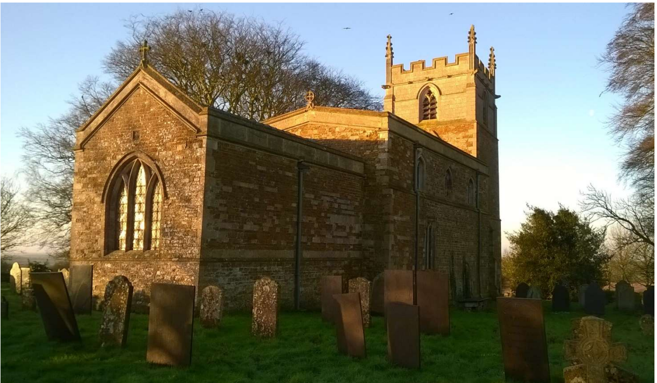
2: The church viewed from the north-east, showing the windowless north wall of the chancel and the single window and blocked door in the north wall of the nave, below the clerestory level. The sparsity of memorials north of the building is also clear
