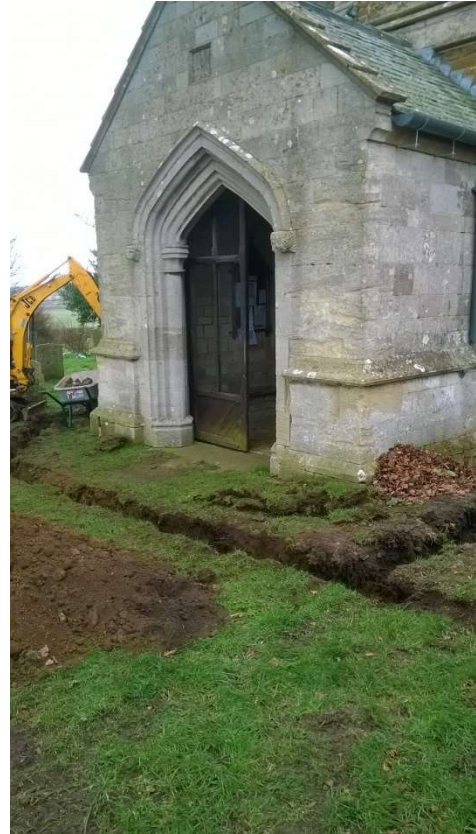
14: The porch during excavation of the trenches, looking north-west
