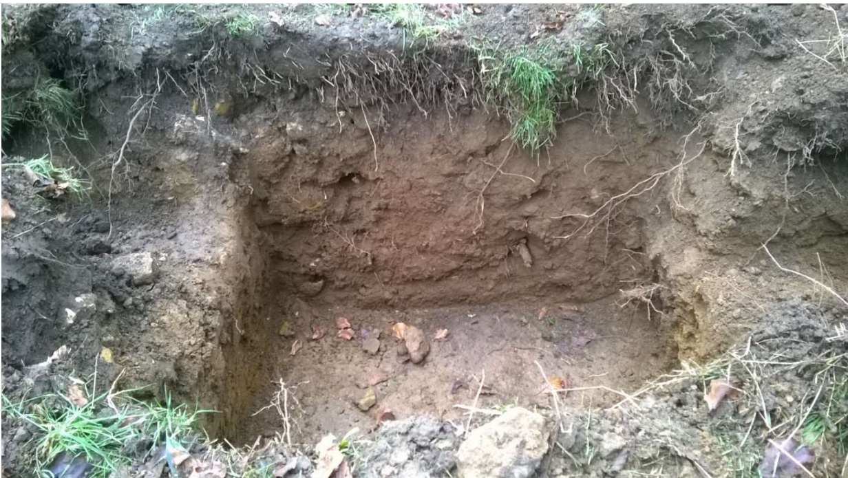
23: Excavated 900mm-deep pit to take silt collection chamber, looking east
