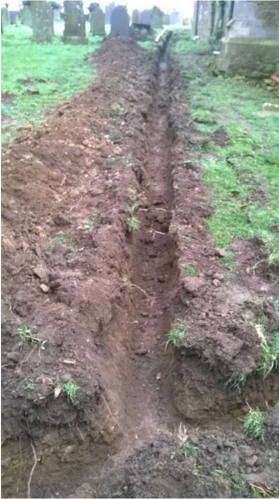
21: Excavated trench along the north side of the church, looking east
