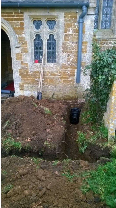
7: Trench for drain from corner of vestry looking north
