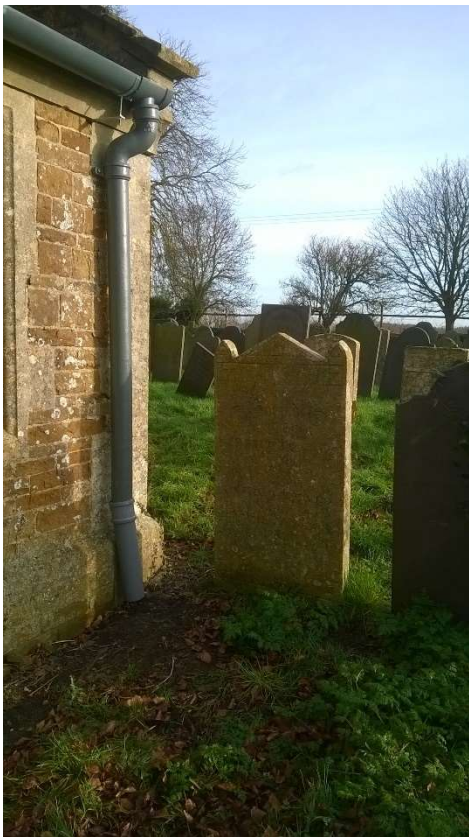
5: The corner of the vestry, showing the closeness of the headstones to the building here, looking north-east
