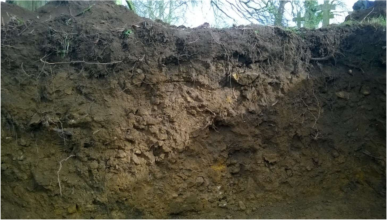
28: West-facing section of 1.10m-deep pit for the soakaway
