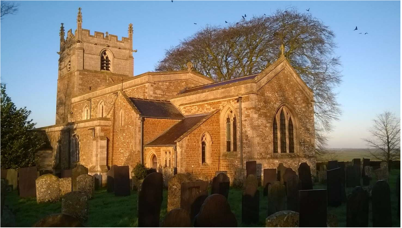
1: The church viewed from the south-east, showing the tower, nave and chancel, with the later additions of the aisle, organ chamber and vestry built onto the south side.
