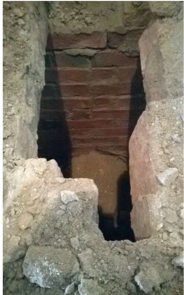
44: Brick vault, looking west, towards the entrance to the tower
