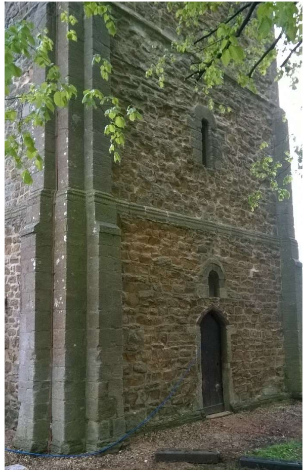
3: West face of the tower
