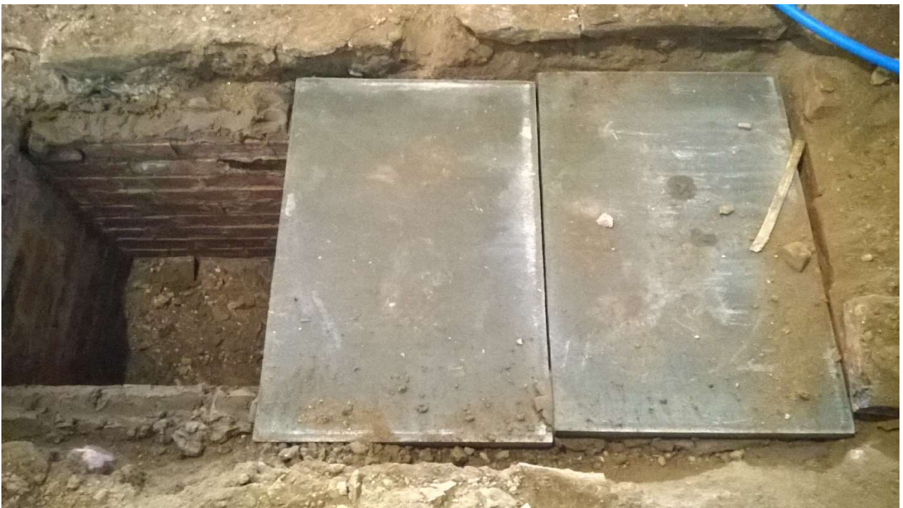
45: Brick vault during capping
