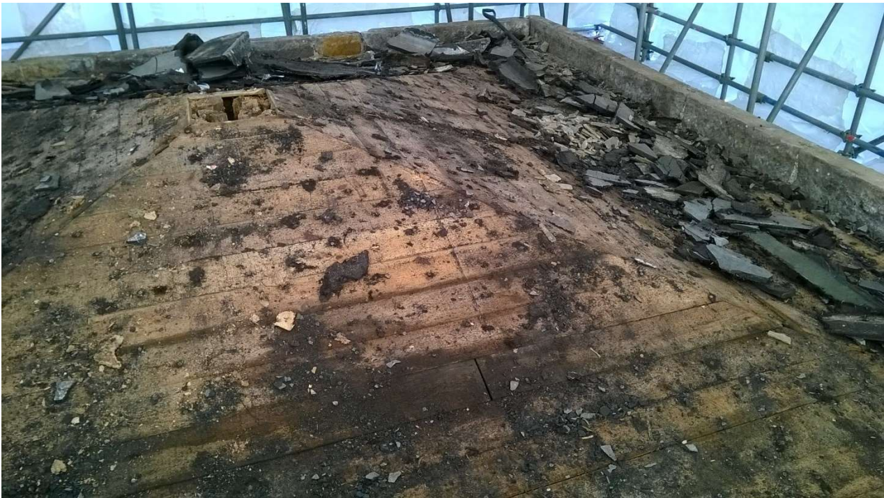
7: The tower roof during removal of the old asphalt layer
