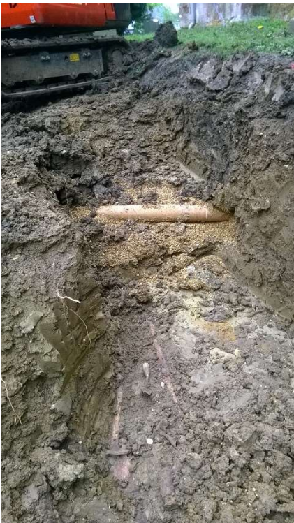
24: Skeleton truncated from left hip to right thigh by later grave; also showing the drain from the nave to the soakaway pit, looking east
