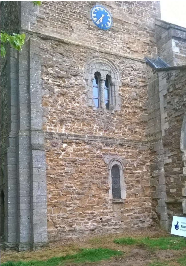
2: South face of the tower
