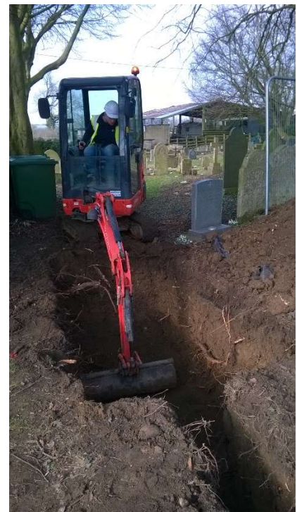
34: Excavating the south-west soakaway pit, between the path and headstones, looking west
