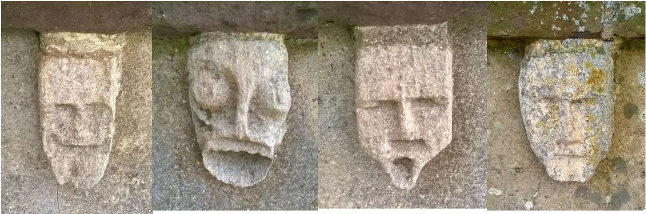
6: Selection of corbels from under the parapet of the tower roof
