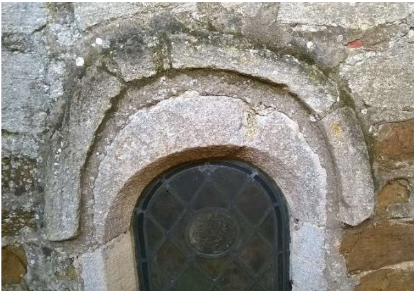
4: Hood-mould of window in lower storey south face of the tower
