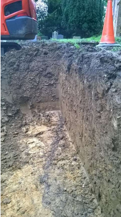
21: Coffin stain in base of the trench arch drain, looking east
