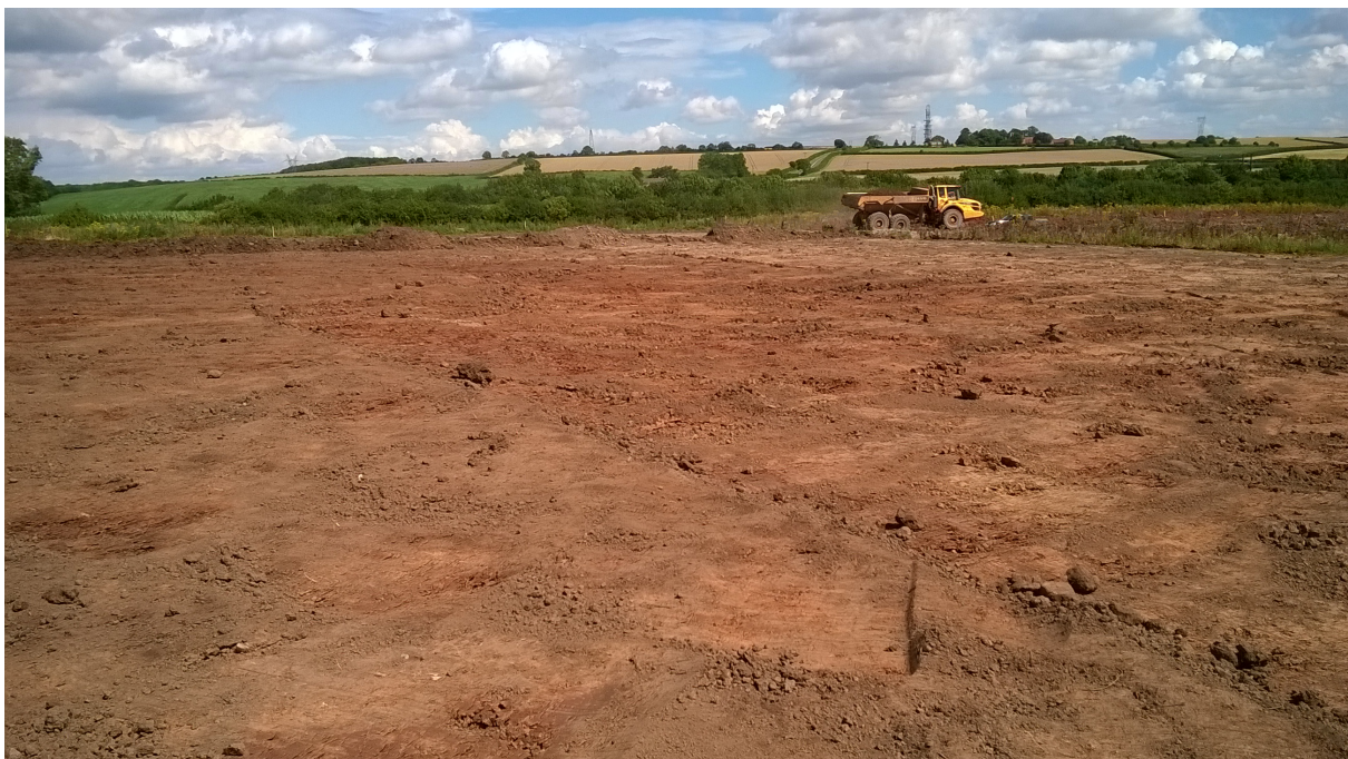
Plate 1: Stripped surface looking north from the former Golden Hill Lane, 1 August 2017
