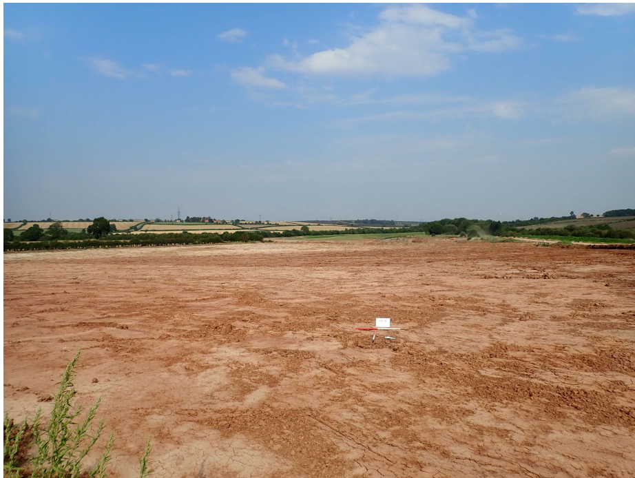
Plate 5: Stripped surface after removal of topsoil, looking north-east
