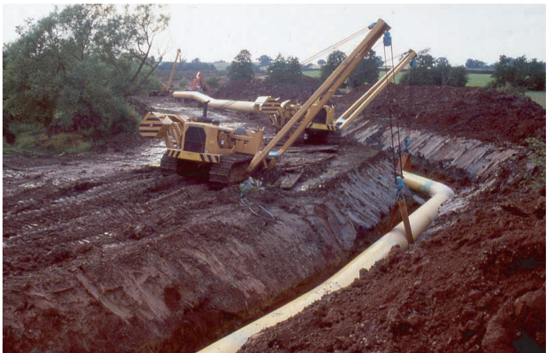
Plate 2: Pipe laying at the River Alne
