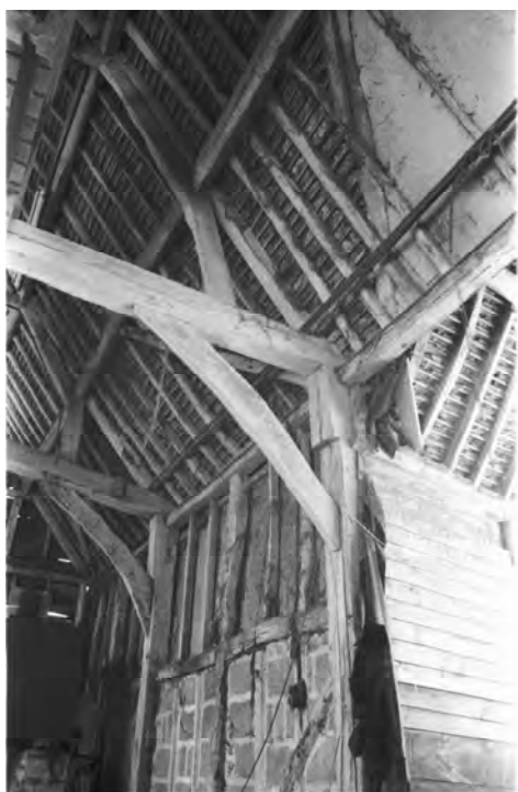
Plate 18. Barn A, detail of truss between bays 2 and 3, looking north-west
