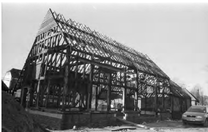
Plate 20. Barn D, looking north-west
