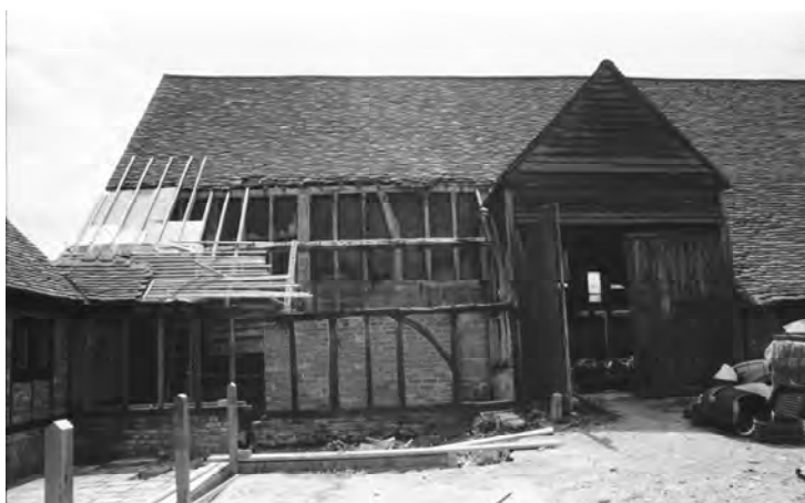
Plate 13. Barn A, west end, looking south-east
