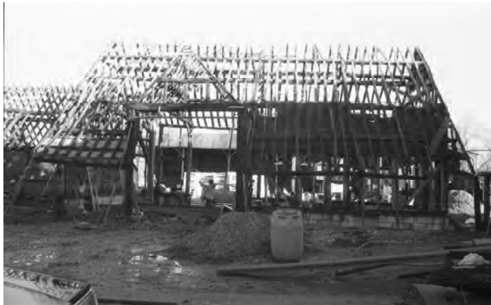
Plate 19. Barn D, west elevation
