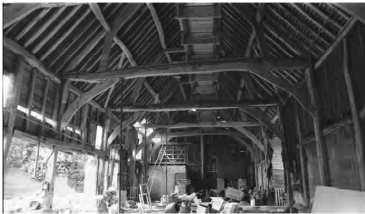
Plate 15. Interior of Barn A, looking south-west
