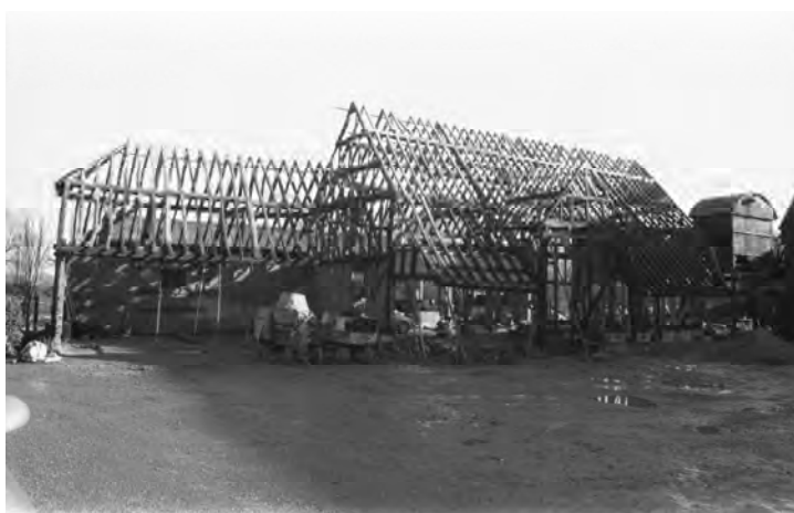
Plate 21. Barn D and Barn F, looking south-east
