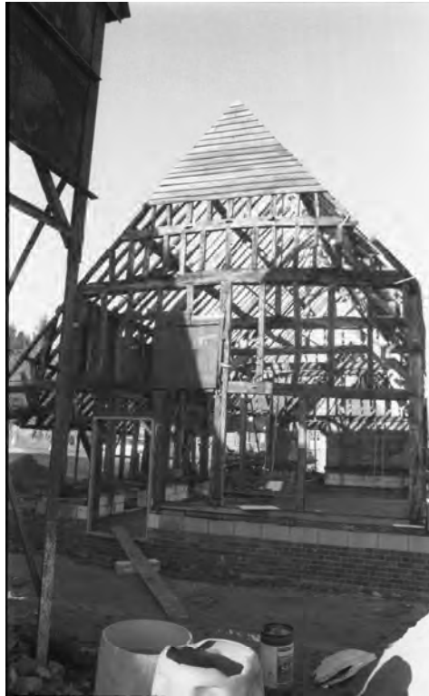
Plate 22. Barn D south elevation
