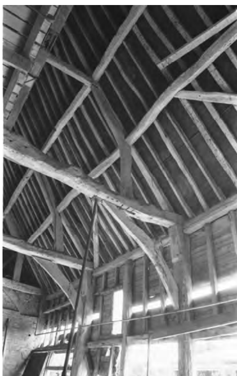
Plate 17. Barn A, detail of truss between bays 4 and 5, looking south-east
