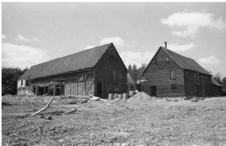
Plate 12. Barns A and D, looking north-west
