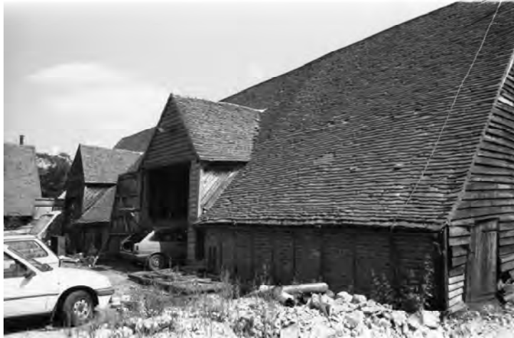
Plate 14. Barn A, east end, looking south-east
