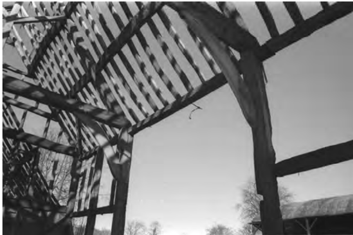
Plate 24. Barn D, detail of trusses between bays 2 and 3, and 3 and 4,
