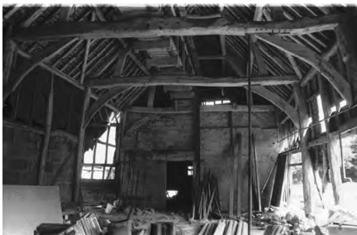
Plate 16. Interior of Barn A, looking north-east
