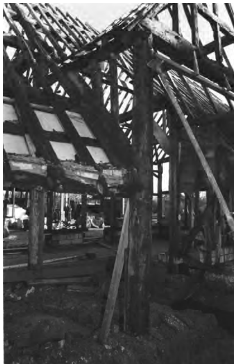
Plate 23. Detail of Barn D entrance, looking south-east
