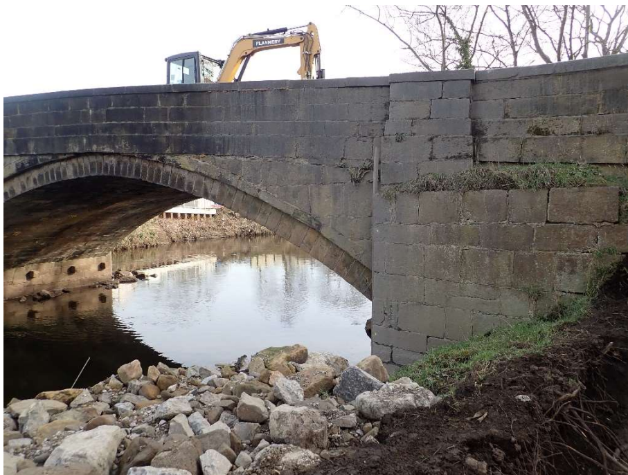
Plate 6: Deck fill excavation, general shot, work in progress.
