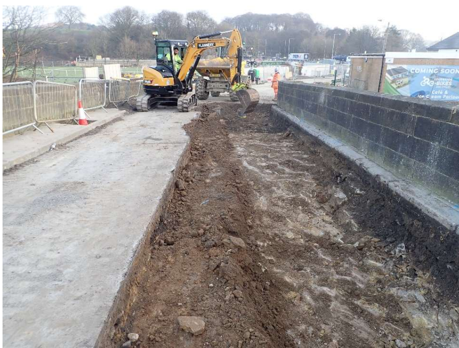
Plate 4: Deck fill excavation, South section, overview of 100004 & 100006, facing east.
