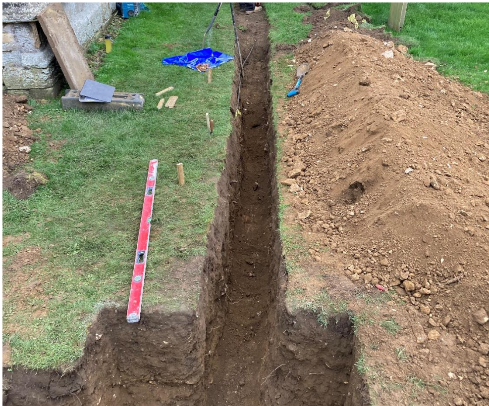
Photograph 8: General view of service trench west of tower, facing south.
