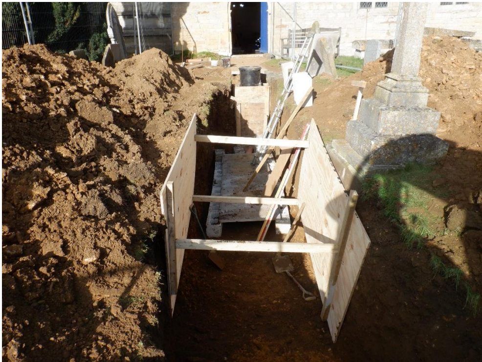
Photograph 40: Completed drainage trench, facing north.
