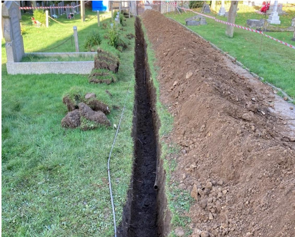
Photograph 1: Service trench to the north of the church, facing north.
