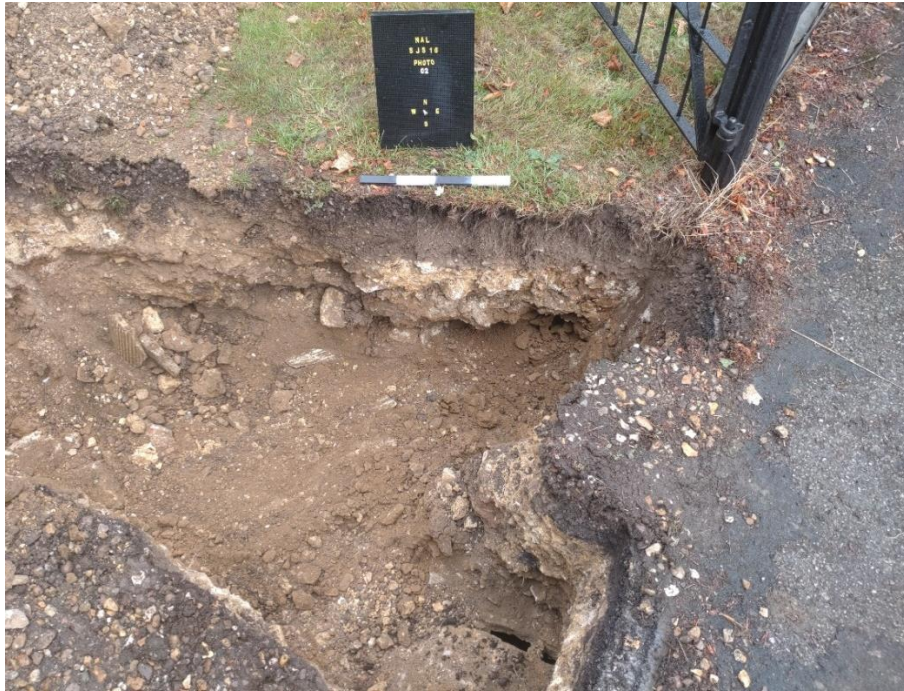
Photograph 1: Cut 04 containing stone topped culvert, facing northeast.
