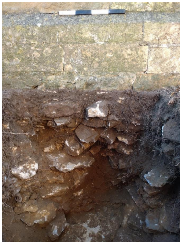
Photograph 6: Tower foundations 16 and 18, facing east.
