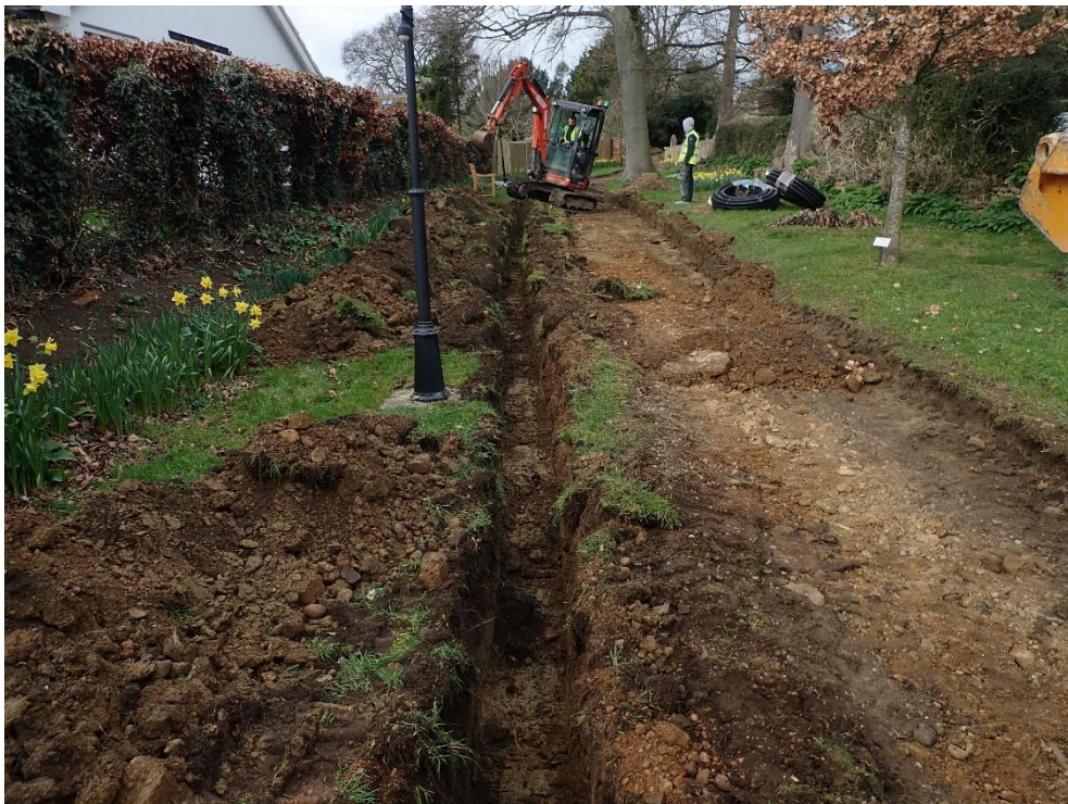
Photograph 9: Excavation of the conduit trench, facing southwest
