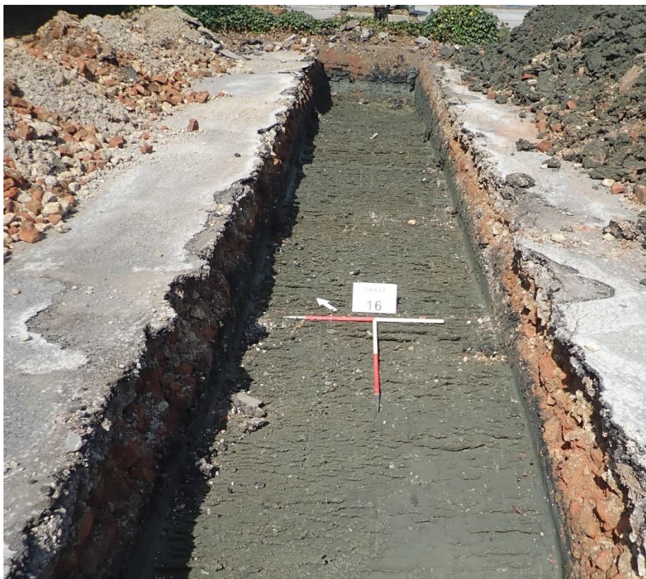
Plate 21: Trench 16, facing north-east.
