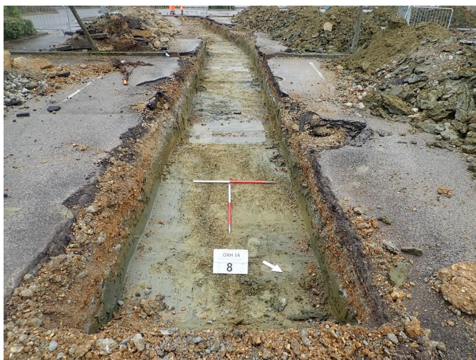
Plate 10: Trench 8, facing south-west.
