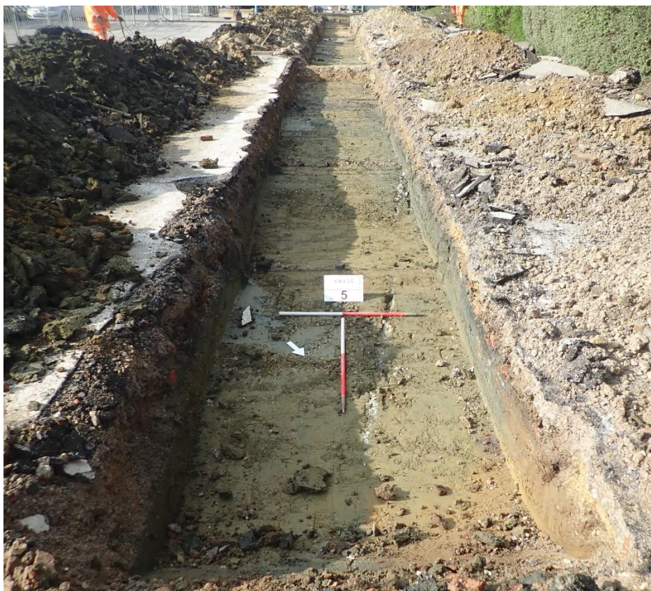
Plate 5: Trench 5, facing south-west.
