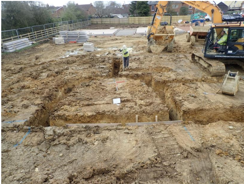
Plate 4: Working shot of house footings
