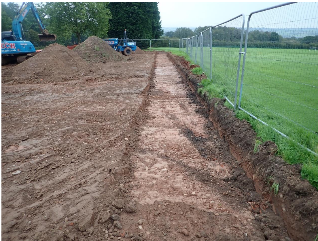
Plate 6: Area 2 under excavation
