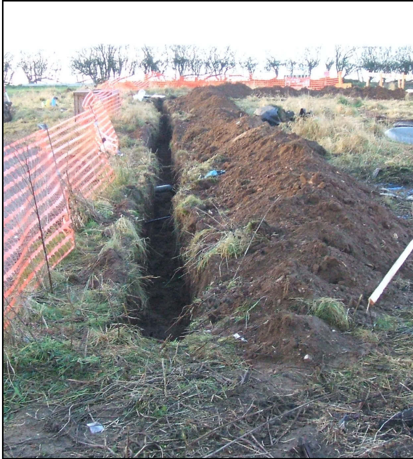
Plate 2: The cable trench, camera facing west
