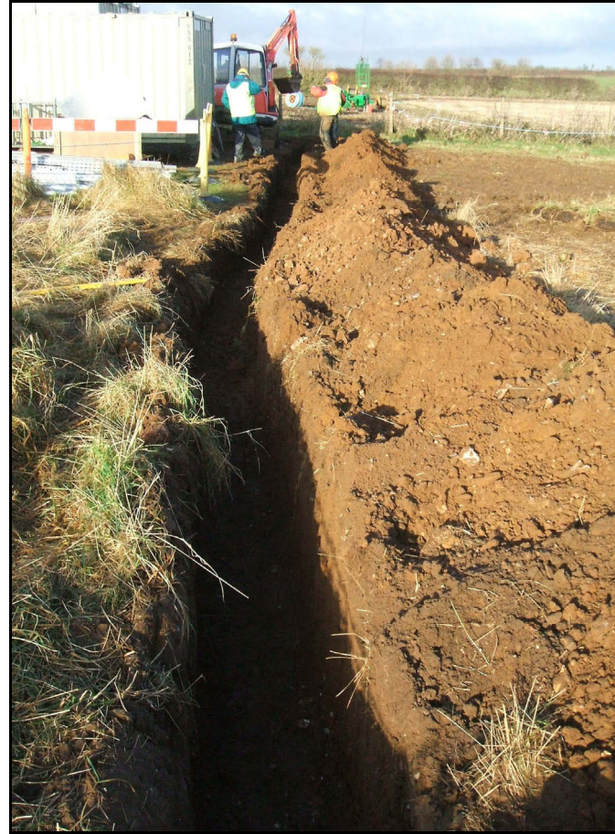
Plate 3: The cable trench, camera facing north
