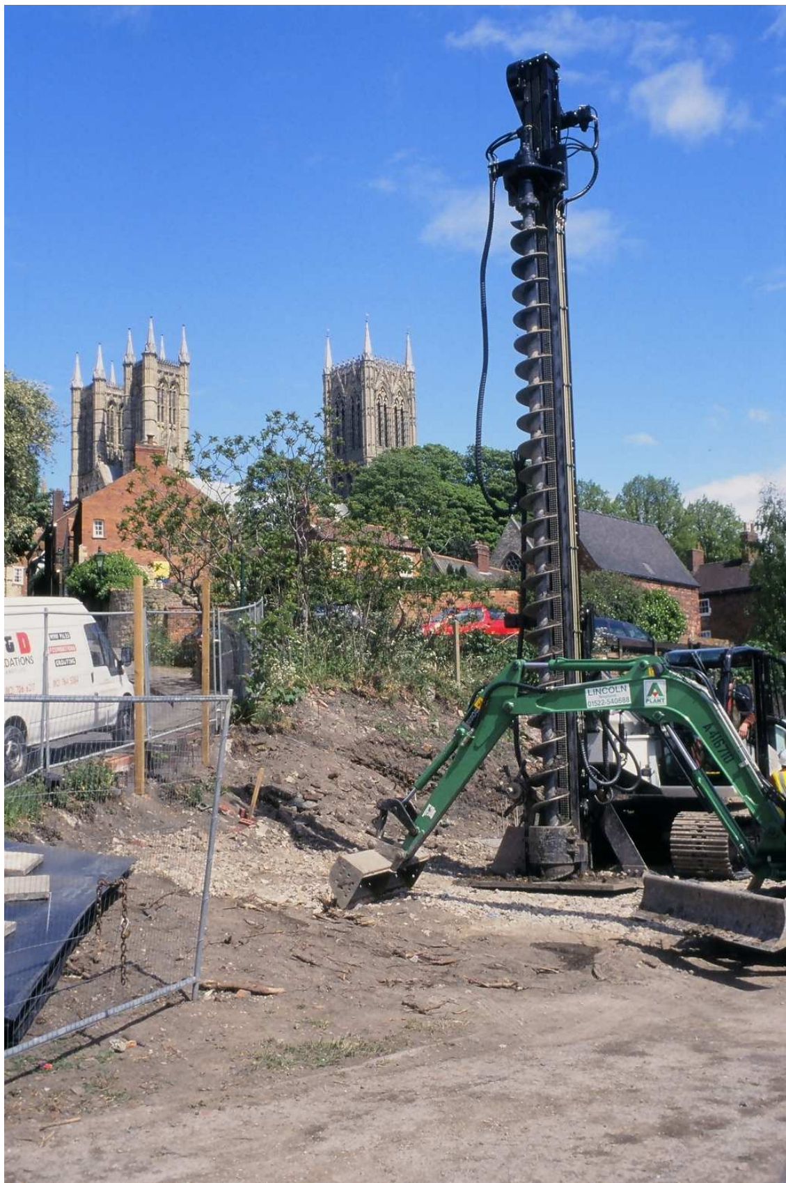
Plate 7 Drilling for piled foundations
