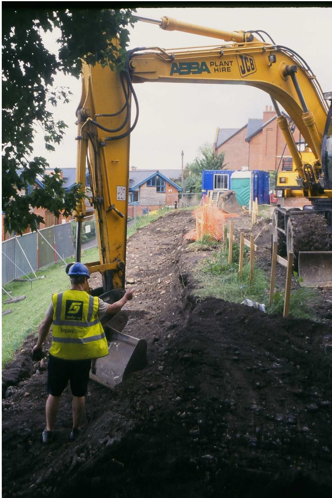
Plate 8 Excavation of the southern terrace bank reinforcement
