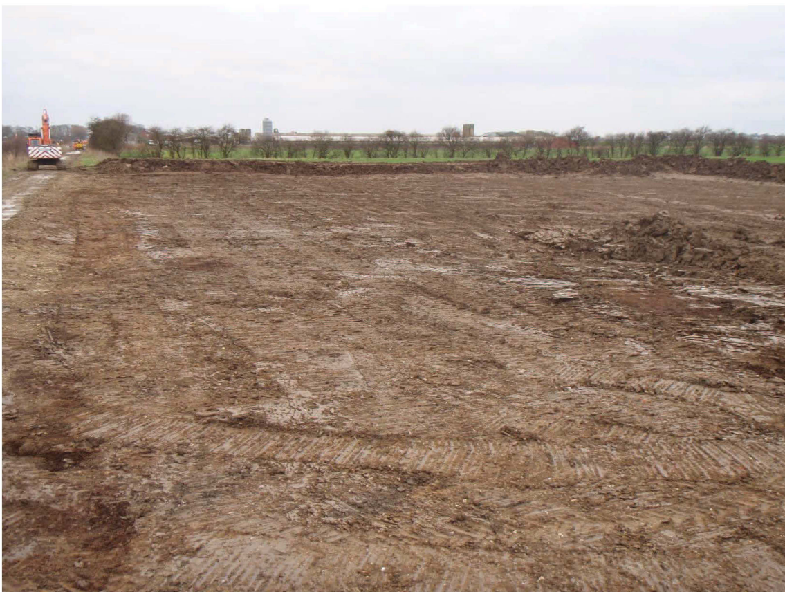
Plate 4: Stripped site compound area, looking north-west.
