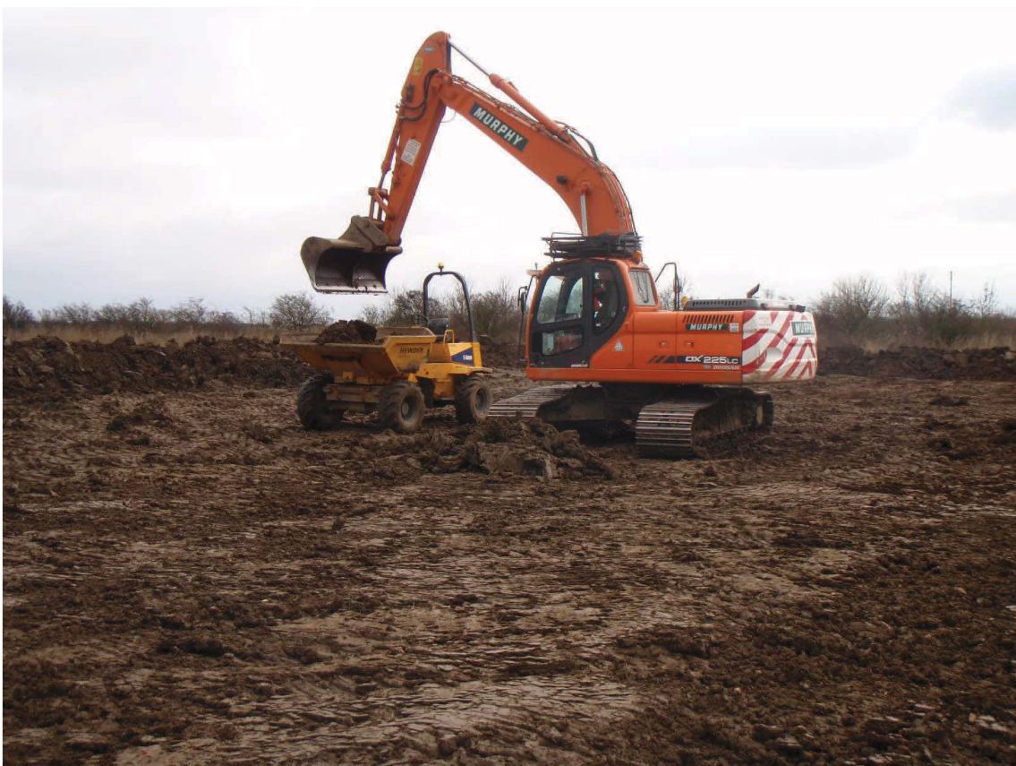
Plate 2: Topsoil strip working shot.
