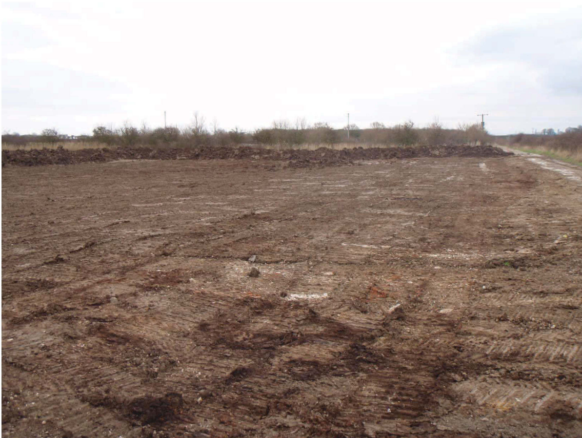
Plate 3: Stripped site compound area, looking south-east.
