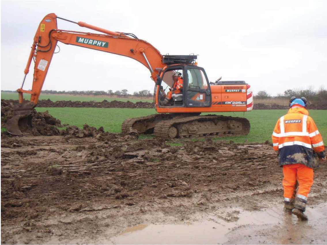
Plate 1: Initial topsoil strip working shot.
