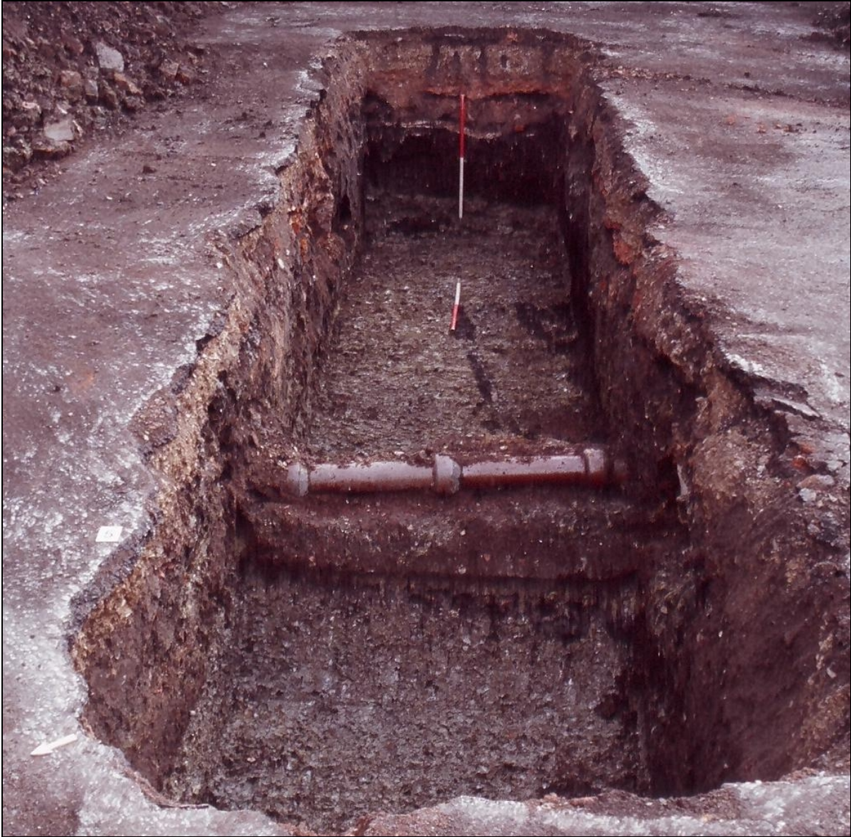
Plate 15: Trench 5 following second phase of machining. Camera facing south east
