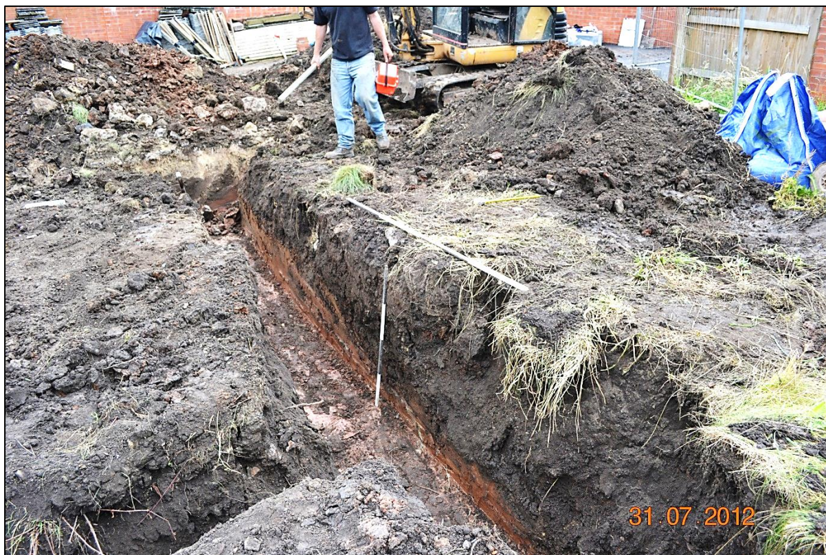
Plate 2: Part of western foundation trench, facing SSW, showing fall in original ground surface from south to north, natural overlain by undifferentiated topsoil context 2/3. The disturbance in the bottom right of the photo is the edge of the land drain. Scales 2 m and 1 m.
