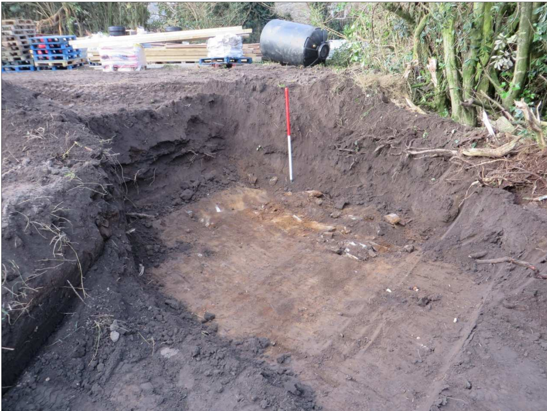
Figure 6 Septic tank pit following stripping to ram (context 9)
