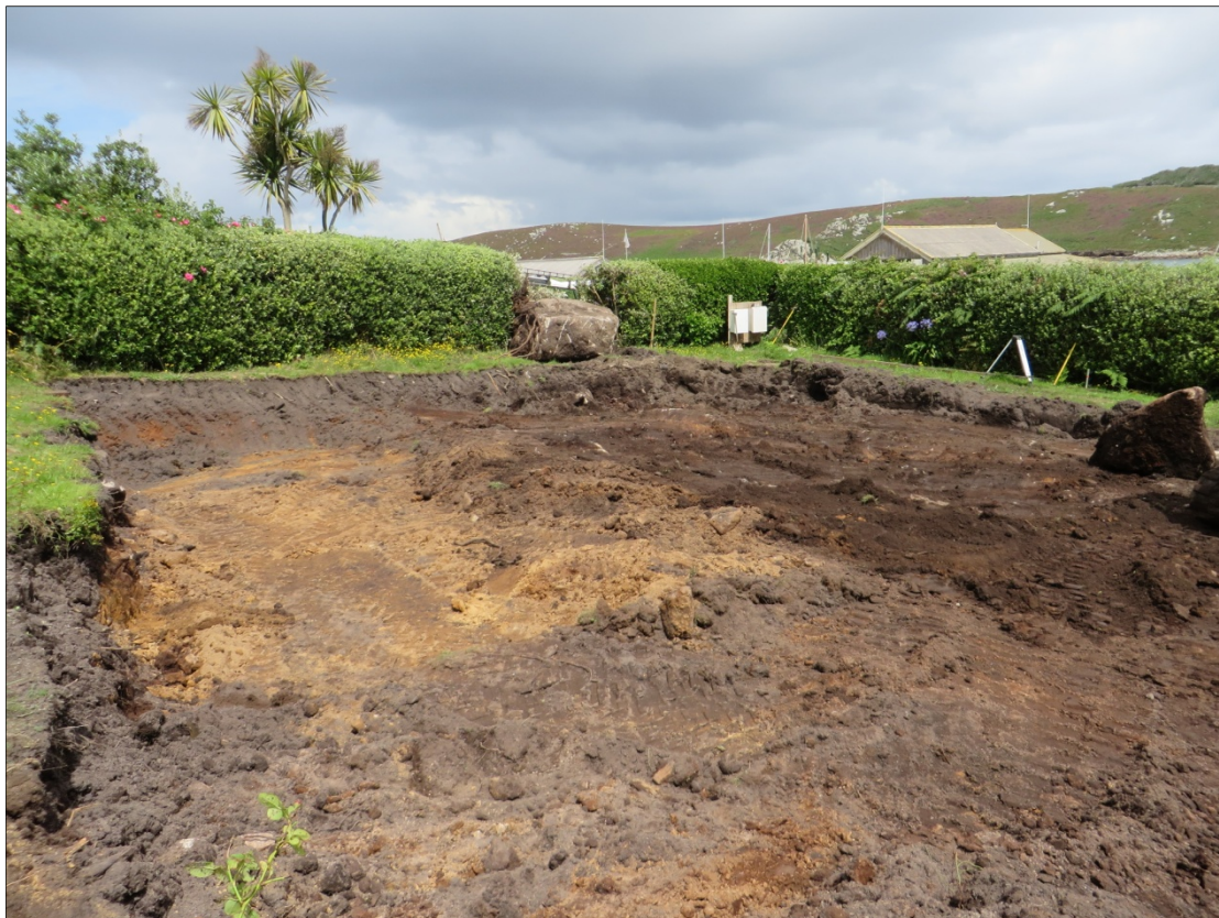
Figure 4 Site of new building following stripping
