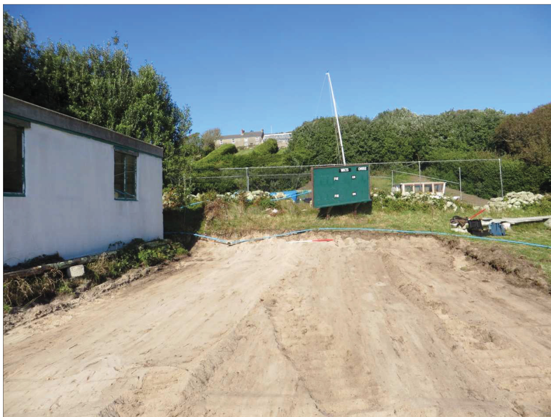
Figure 4 Site after clearing
