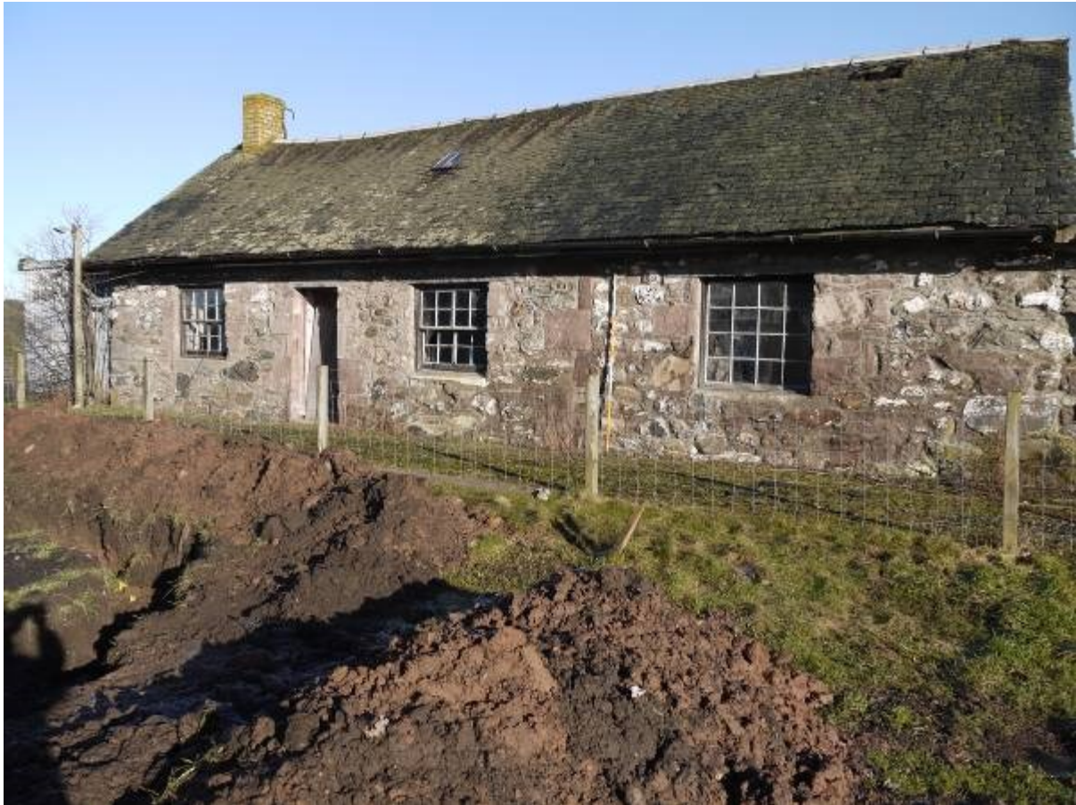
Illustration 9 Southern elevation of main Smithy building (B and C) showing windows, internally blocked doorway and visible straight butt joint to left of scale
