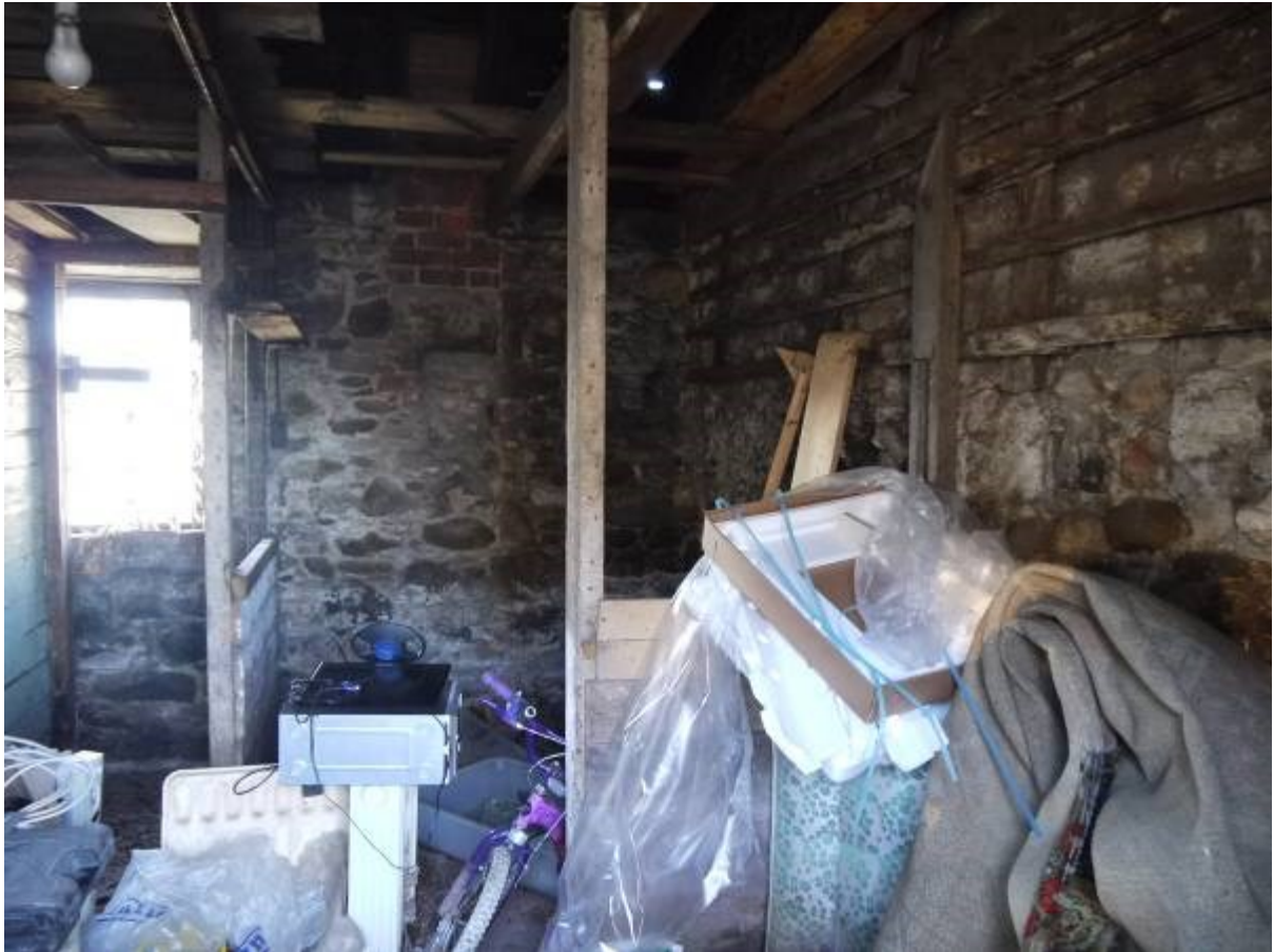
Illustration 17 Interior of eastern room (B) in main Smithy building
