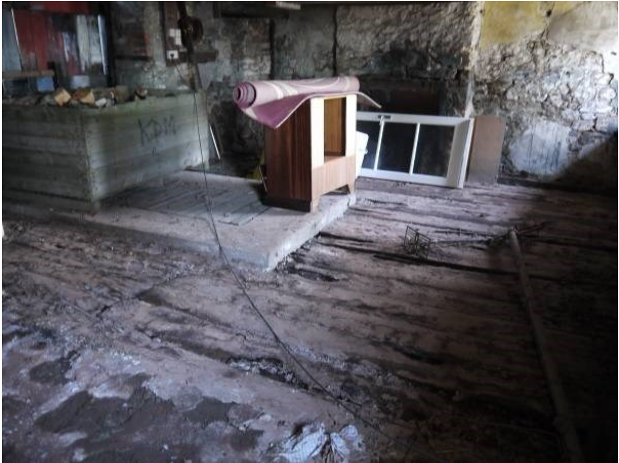
Illustration 19 Interior of western room (C) showing sleeper floor, raised platform and concrete floor in foreground
