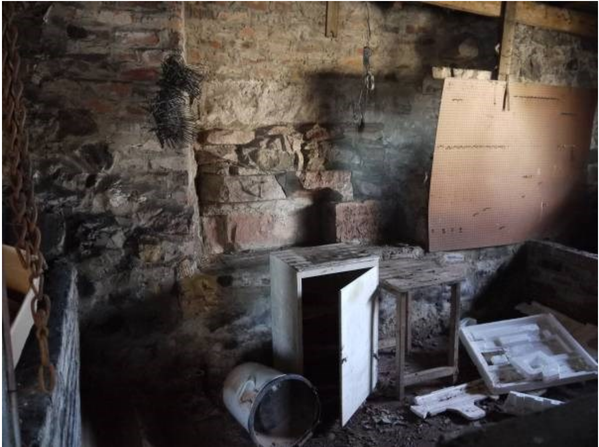
Illustration 15 Interior of Eastern extension (A) showing inside face of blocked window/access point in elevation
