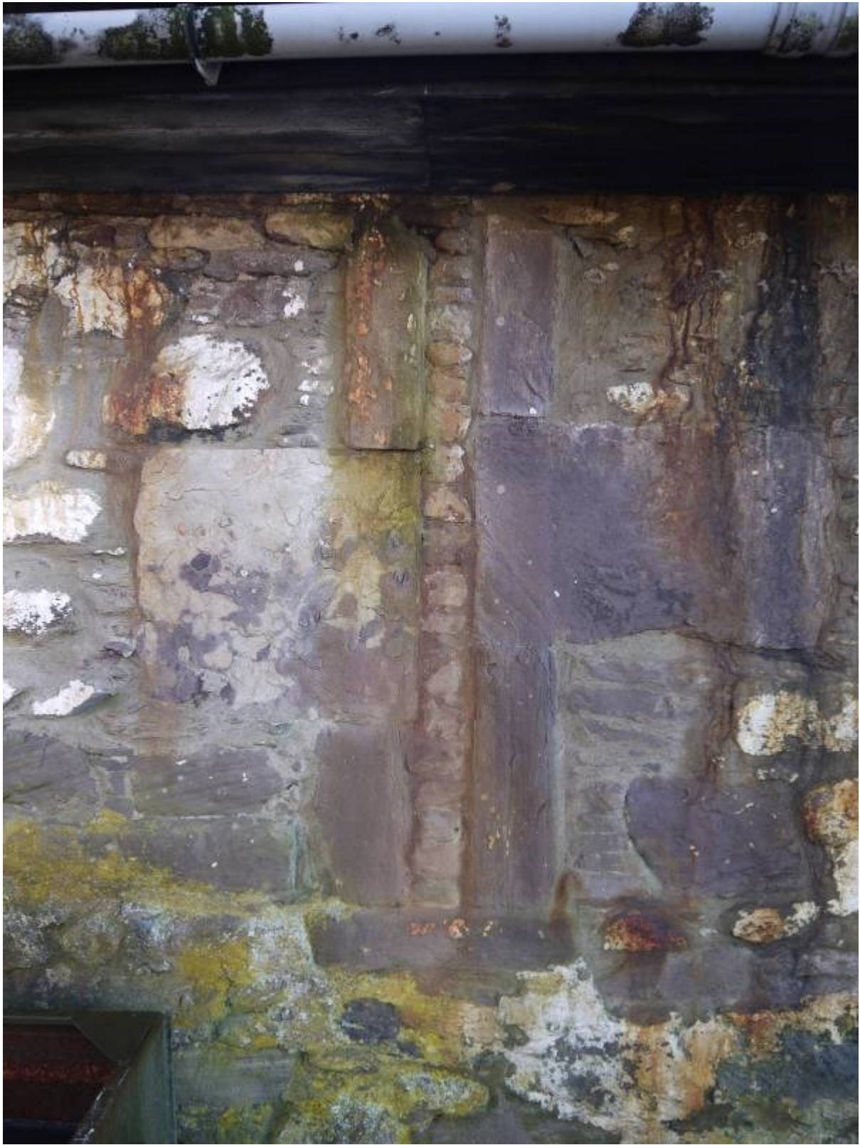
Illustration 14 Blocked slit window in Northern elevation (3 on Illustration 3)
