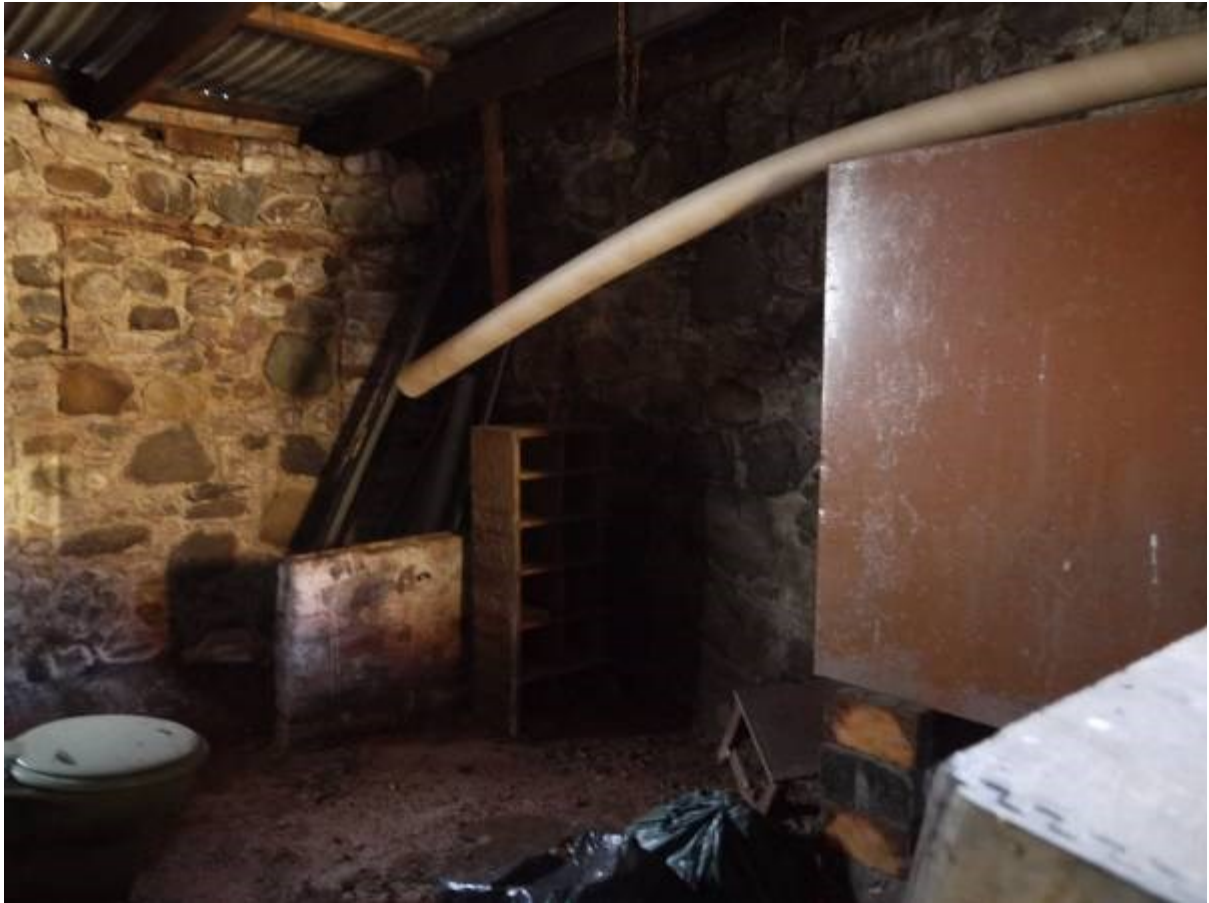
Illustration 16 Northern side of interior of eastern extension (A) showing low subdividing brick wall
