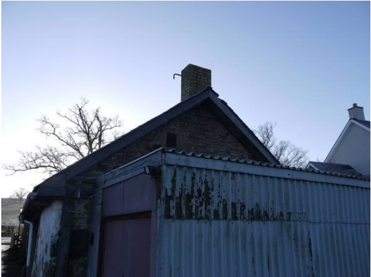
Illustration 10 Western elevation of main Smithy building with extension (D) visible in foreground, small hole/window visible in gable end and brick chimney set back from top of gable
