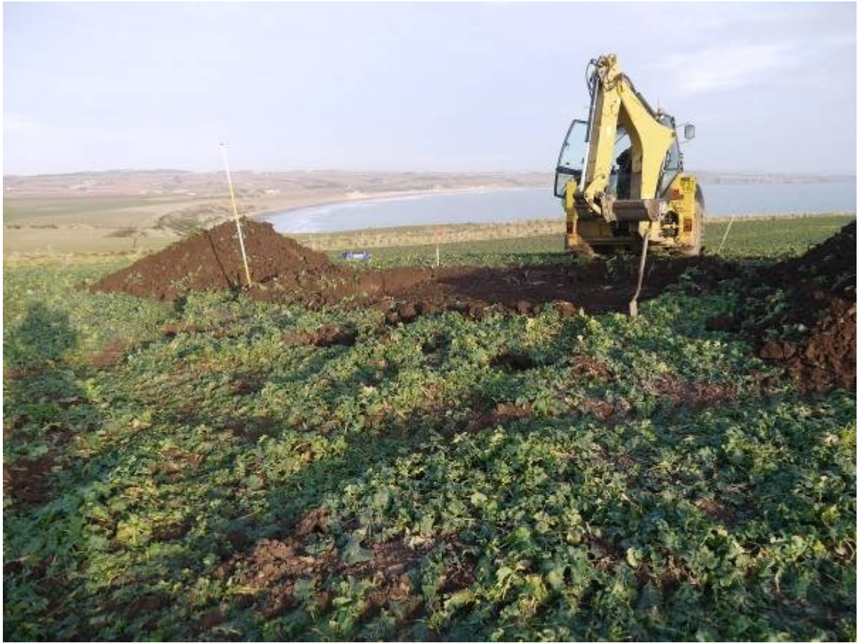
Illus 5 location of stripped area for Turbine 1 looking North
