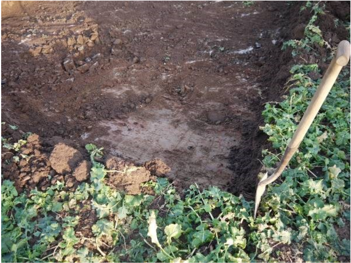
Illus 7 Stripped area for Turbine 1 detailed view of natural clay
