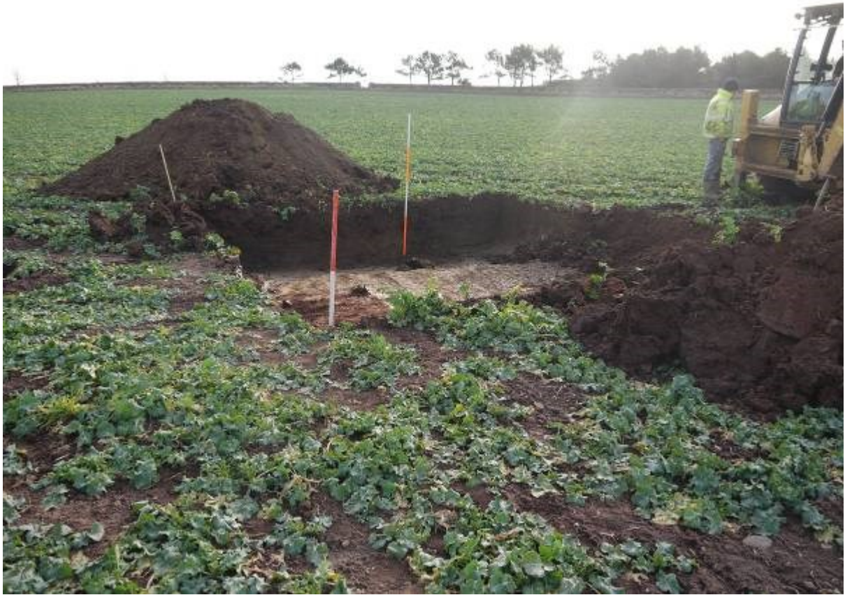
Illus 8 Location of stripped area for Turbine 2 looking South East
