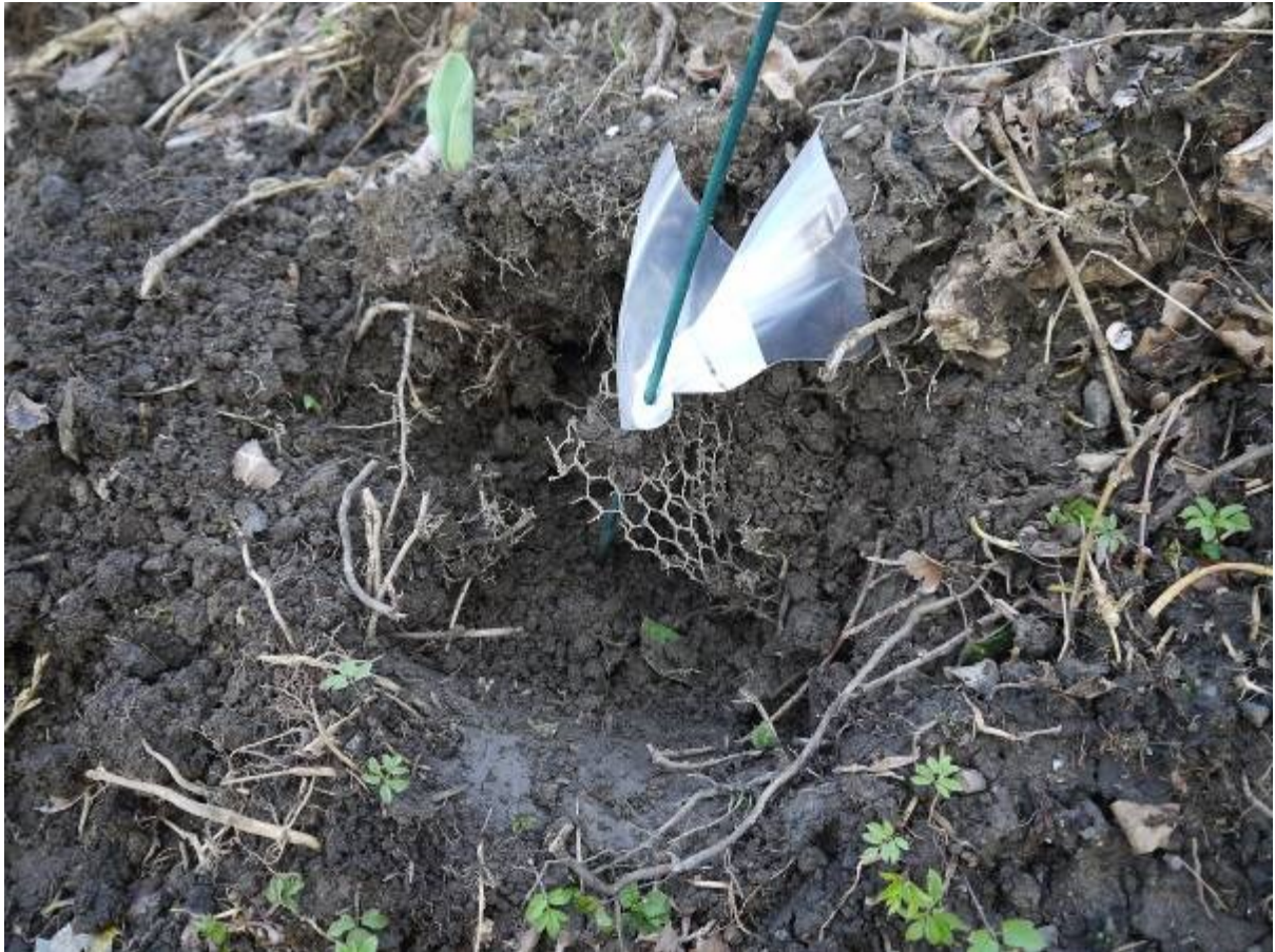
Illus 11 Detail view of layer of chicken wire encountered just below ground surface
