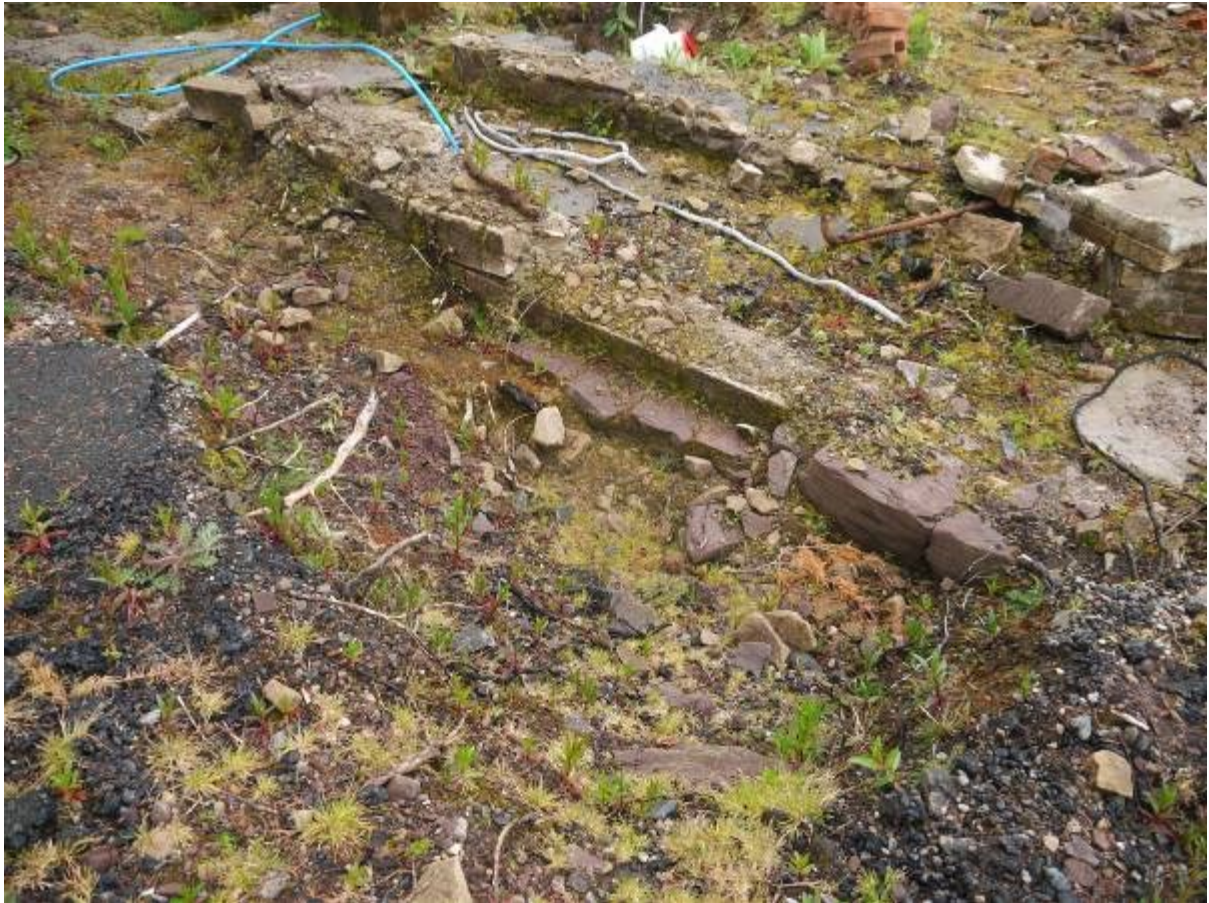
Illus 6 Visible foundations of front of Inverardoch House to South of house plot.
