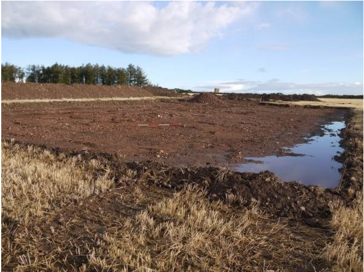
Illus 30 Crane pad for turbine 9 showing natural ground surface
