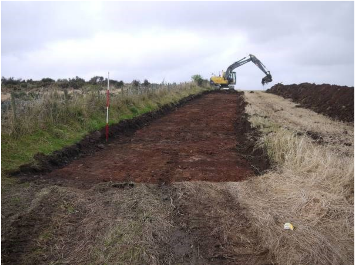
Illus 32 Access track to turbine 7 showing natural ground surface looking West
