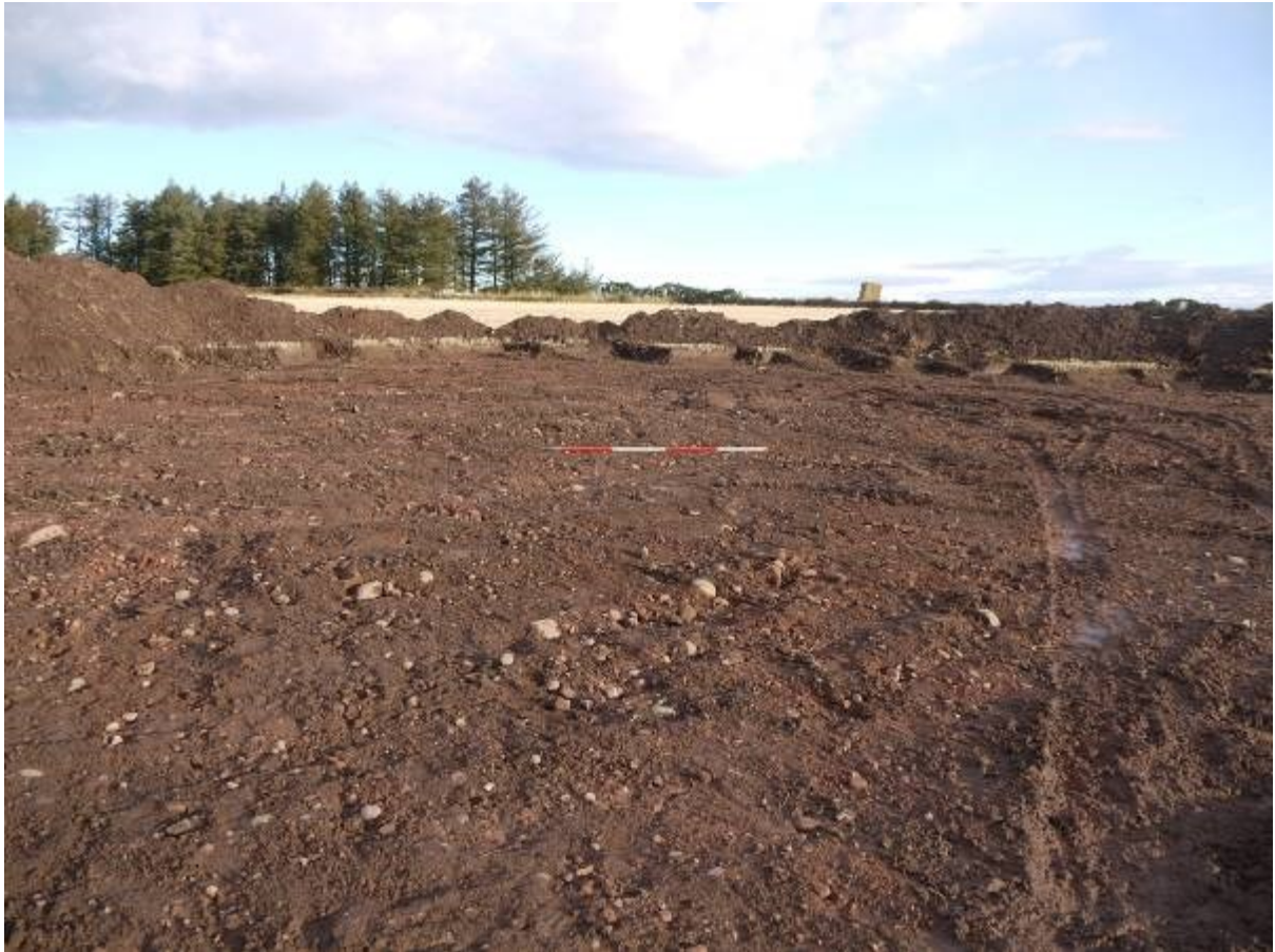
Illus 31 Turbine base 9 showing natural ground surface
