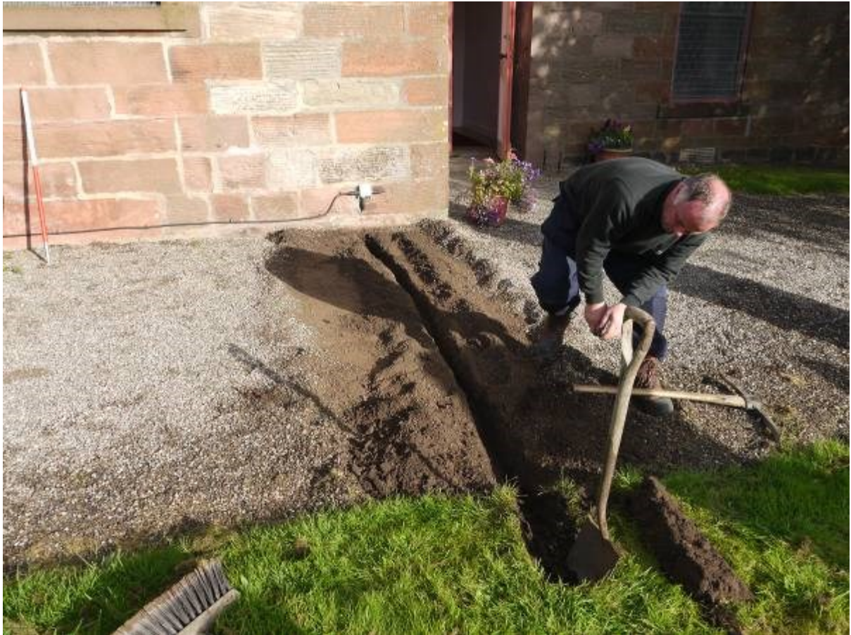
Illus 7 Trench for cable to floodlight 2 looking North (B on illus 3)
