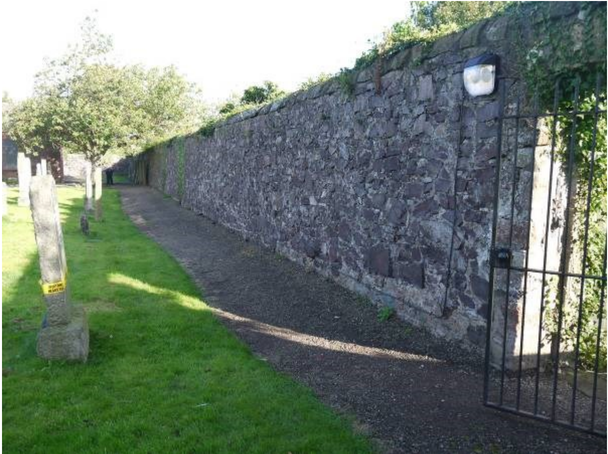
Illus 8 Cable for bulkhead light attached to face of eastern graveyard wall looking north
