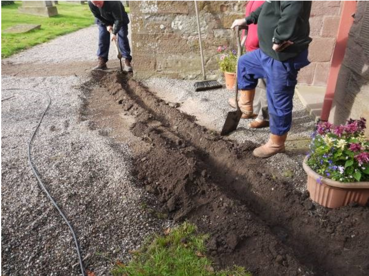
Illus 11 Excavated trench for bulkhead light cable (D on illus 3)
