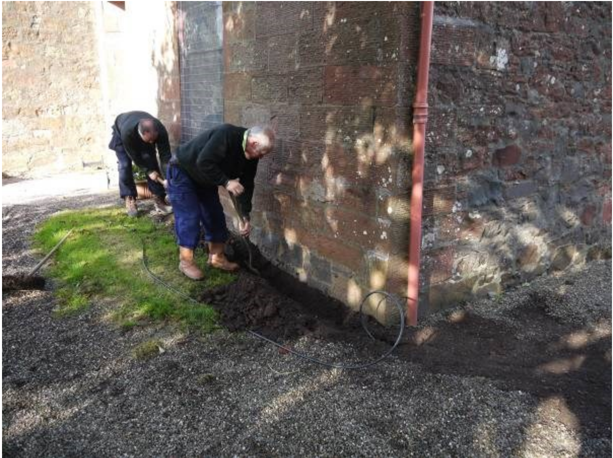
Illus 10 Trench for bulkhead light cable under excavation
