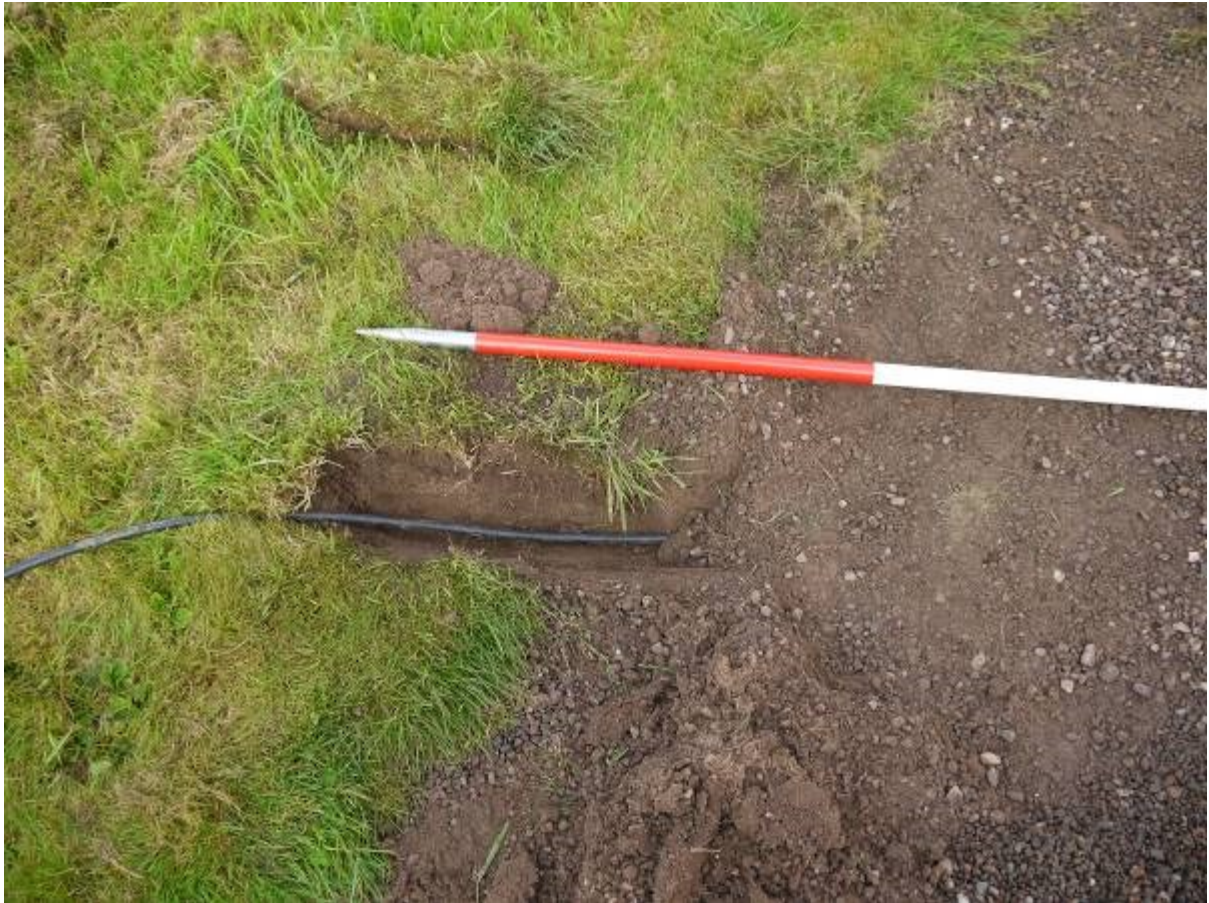
Illus 6 Trench for cable to floodlight 1 looking north (A on Illus 3)
