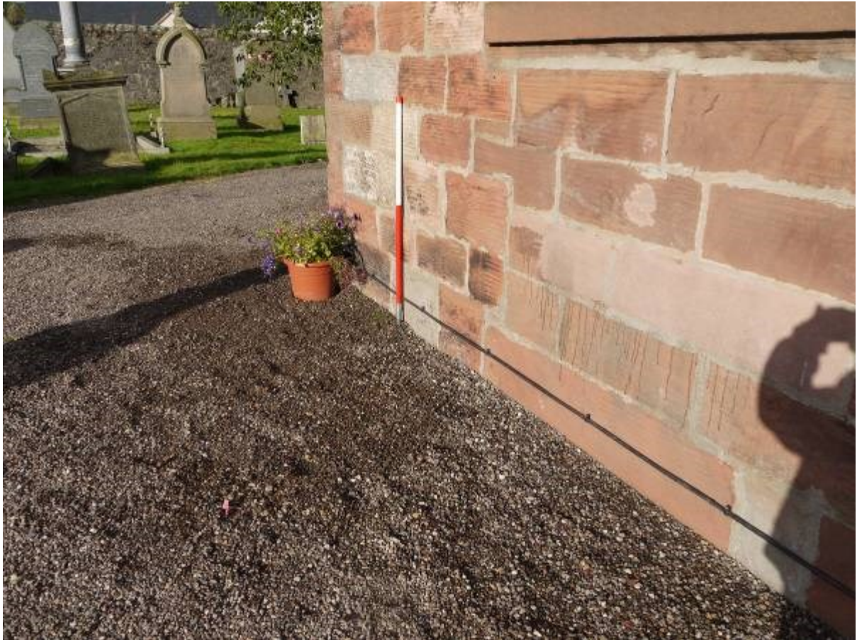
Illus 5 Floodlight cable attached to South wall of Kirk of St Bride looking North West
