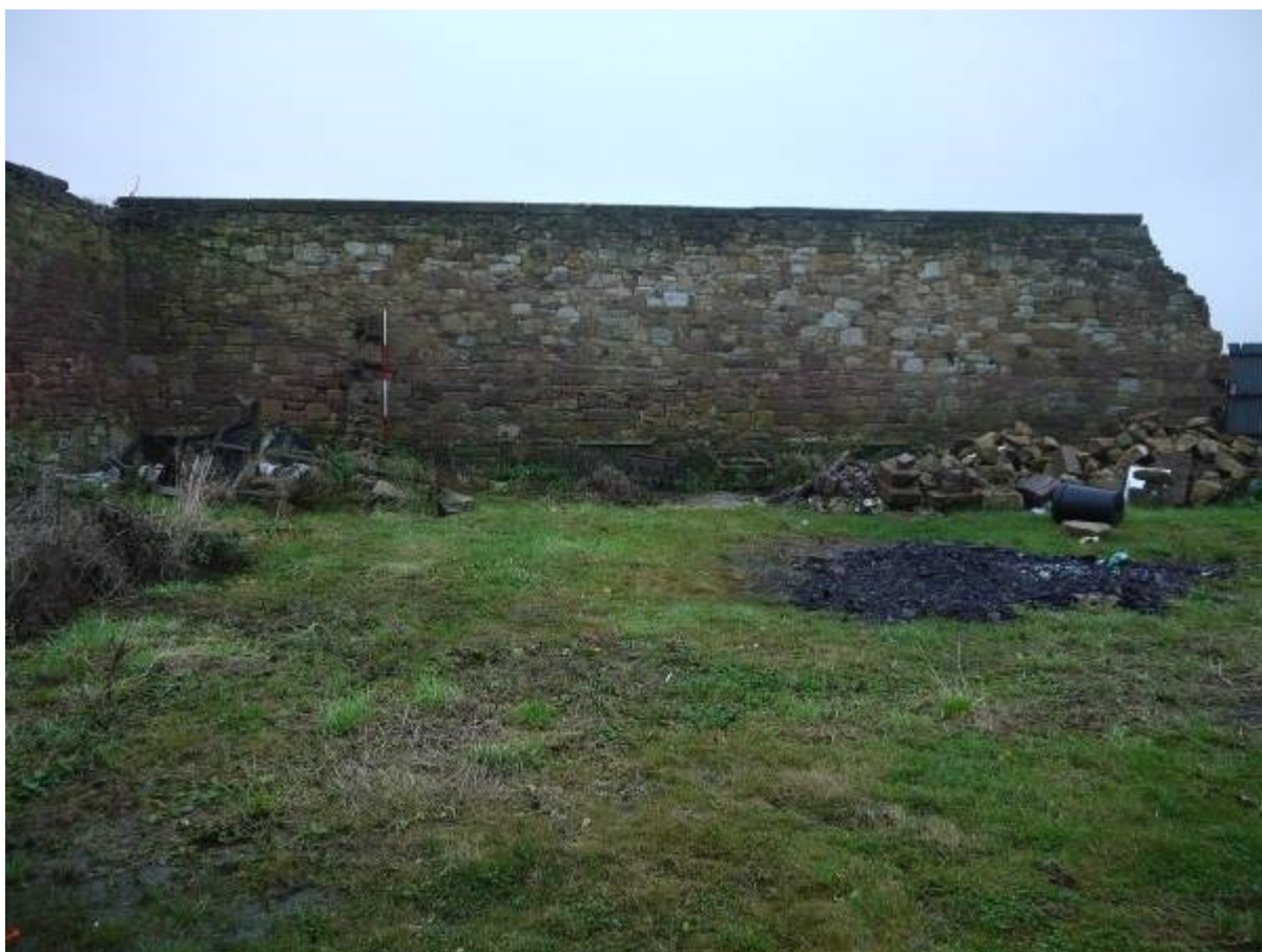
Illustration 37 South Western boundary wall to steading complex with roof raggle of South end of demolished building C (Phase 1) visible beside scale
