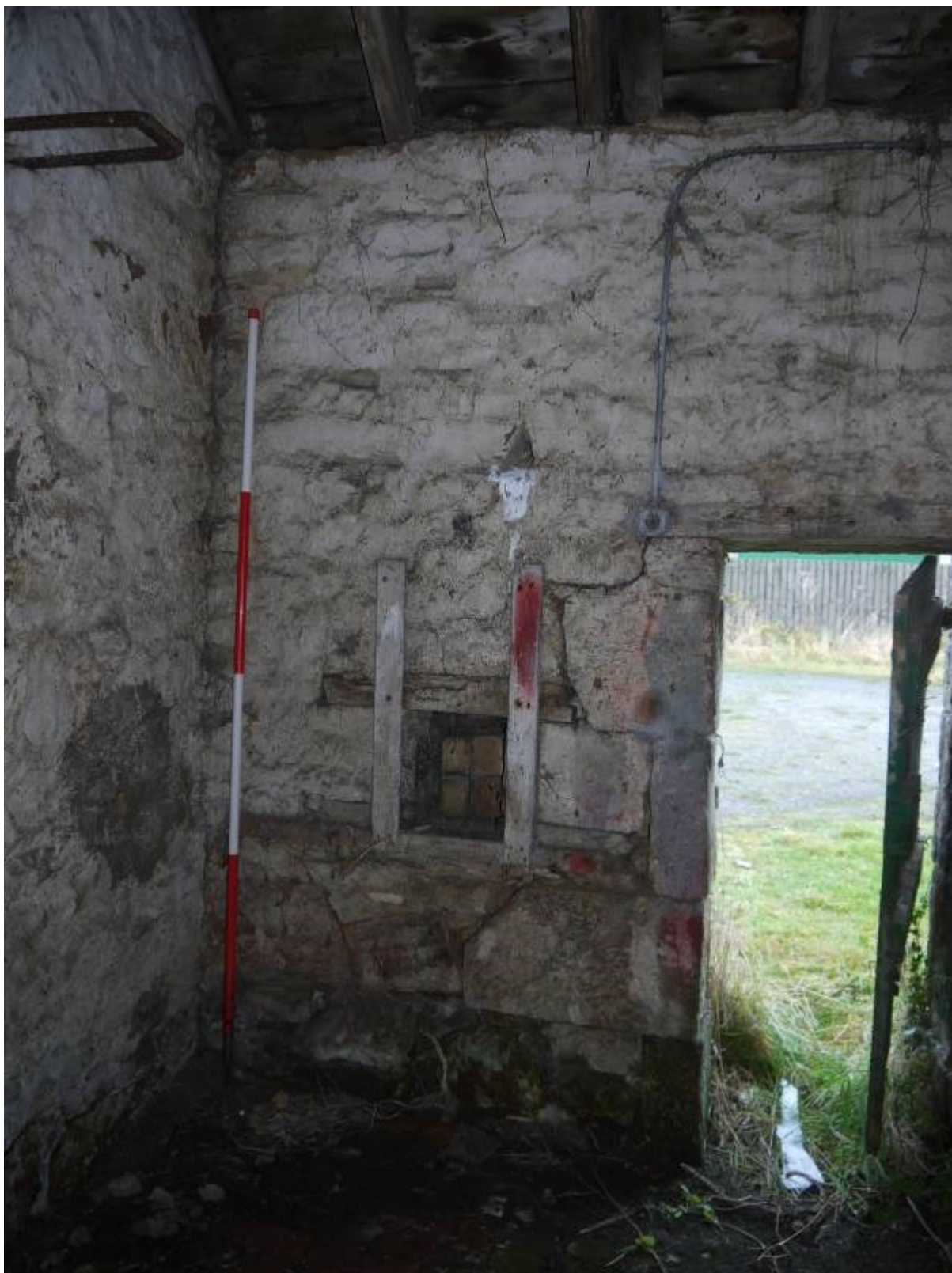
Illustration 24 Blocked hole in North Eastern wall of Room A2 (Phase 3)
