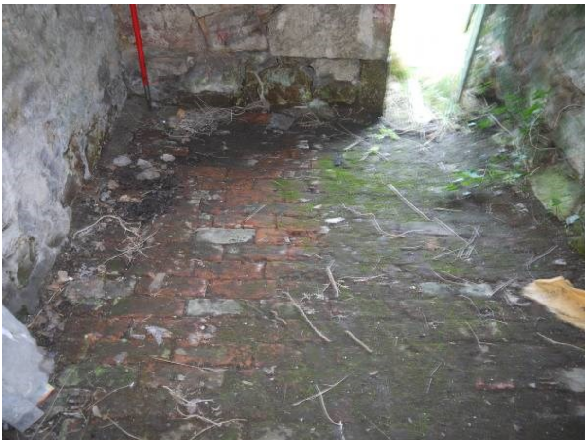
Illustration 25 Brick floor in Room A2 (Phase 3) in Building A
