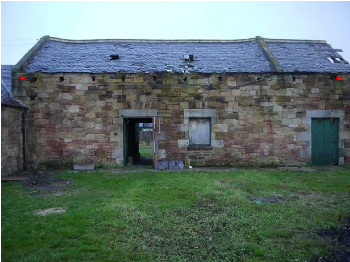
Illustration 26 South West facing elevation of Building B (Phase 1) looking North East, red arrows indicate line of holes just below roof line
