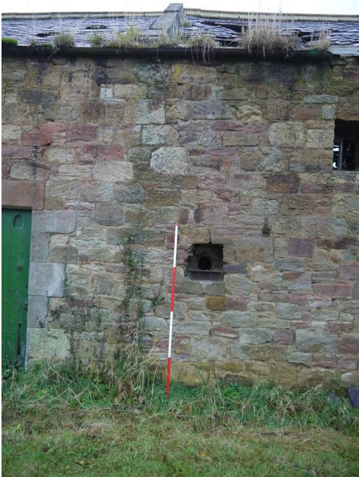
Illustration 17 Small square hole in North Eastern elevation of Building B (Phase 1) providing access to Bamfords Rapid Grinding Rolling Mill looking South West
