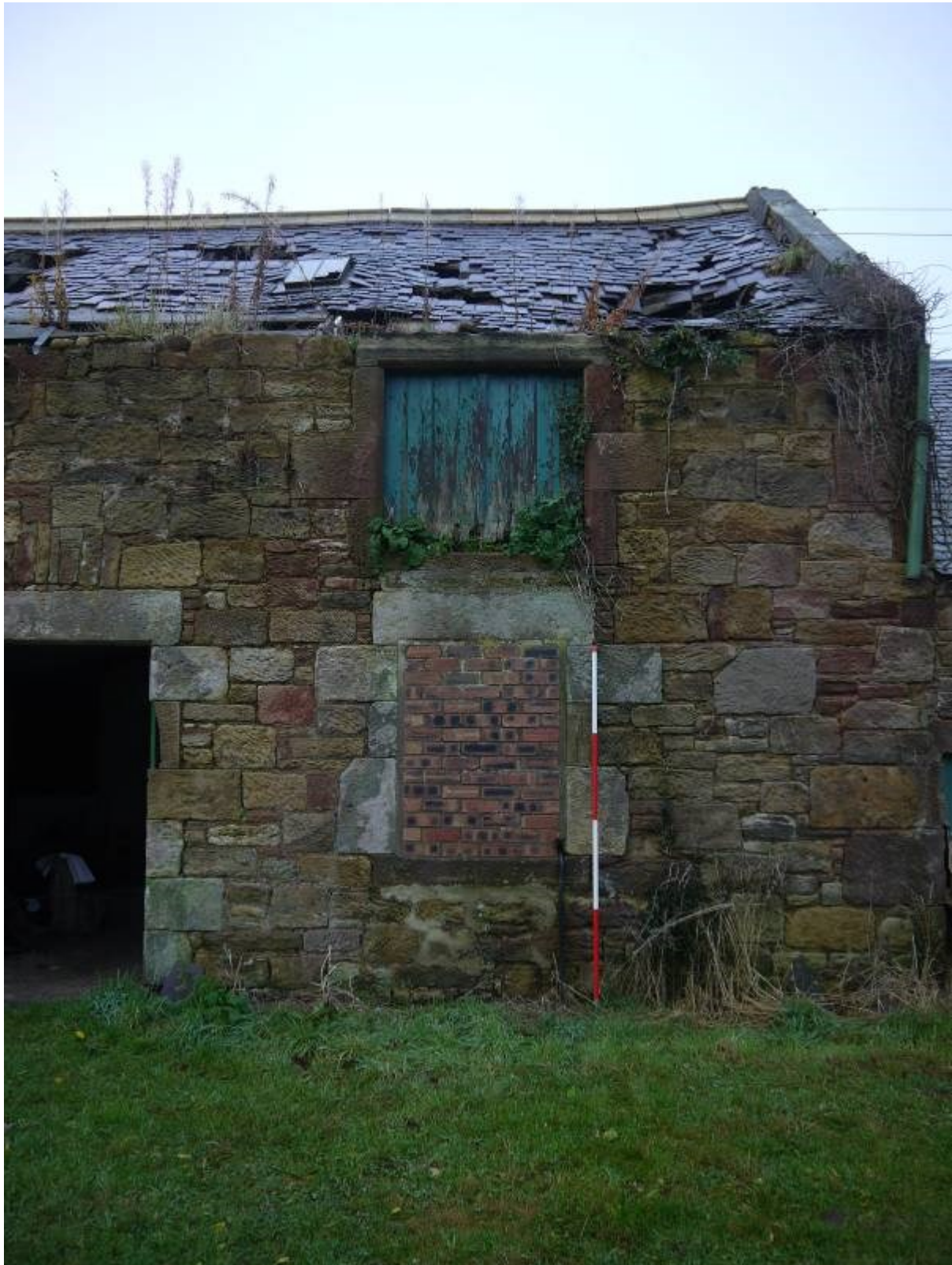
Illustration 15 Northern end of North Eastern elevation of Building B (Phase 1) showing blocked ground floor window and shuttered upstairs window looking South West
