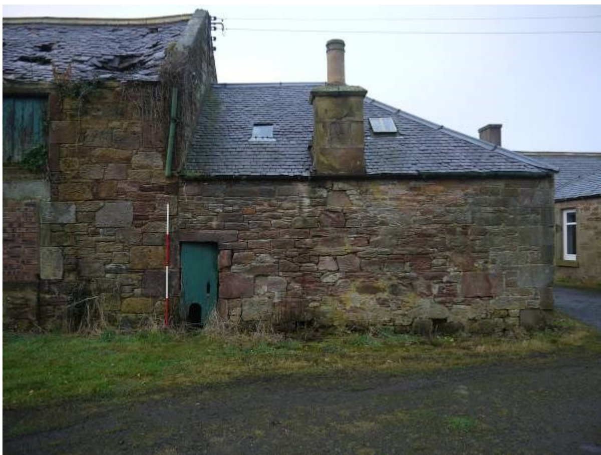
Illustration 14 North Eastern facing elevation of Building A (Phase 2) showing butt joint with building B (Phase 1) and chimney in middle of elevation
