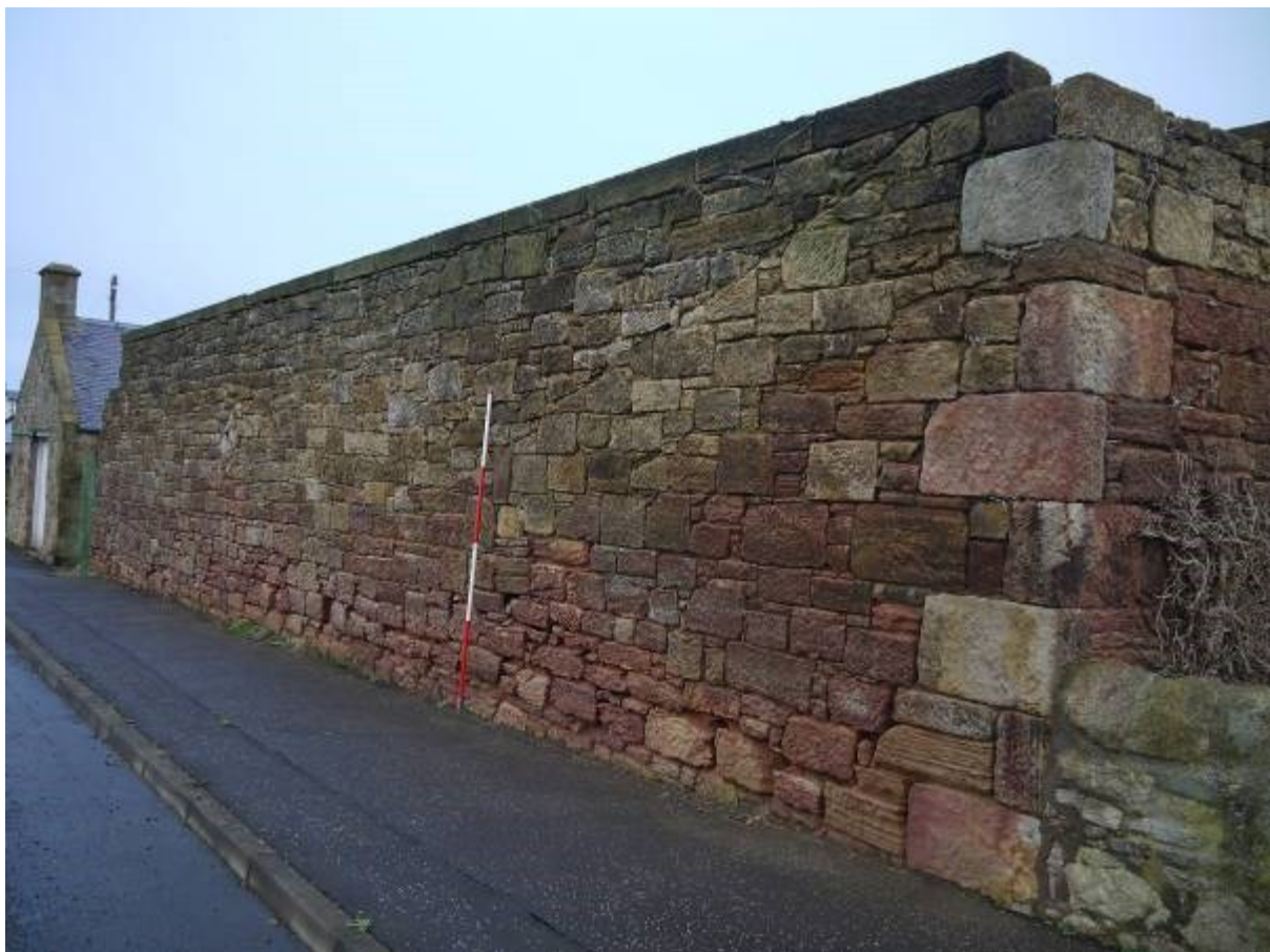
Illustration 8 South West facing elevation of Steading looking North North West, roof raggle visible in wall face gable end of Building A visible in background
