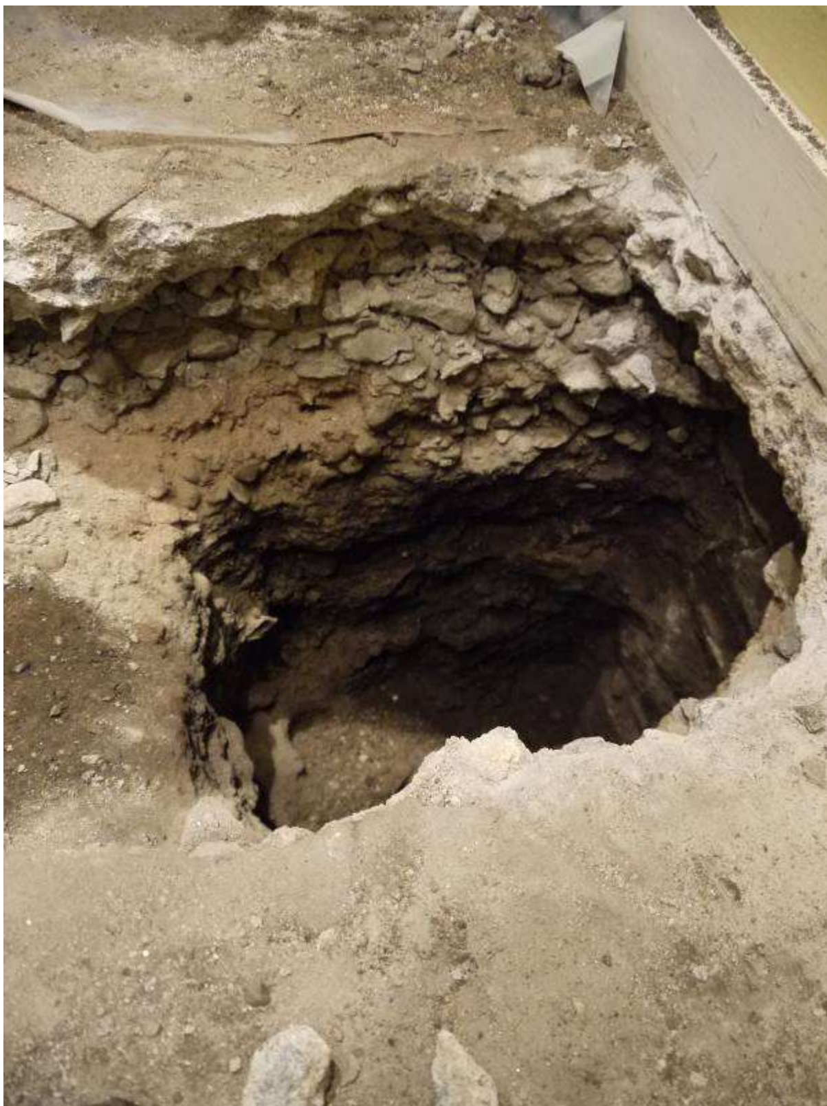
Illustration 26 TP4 excavated to base of wall foundation and natural ground surface looking west
