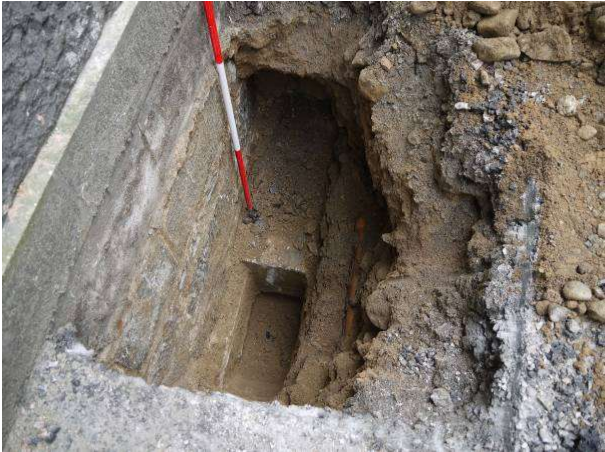
Illustration 29 Machine dug trench against Robert Gordons College in service yard showing deep foundations looking north east
