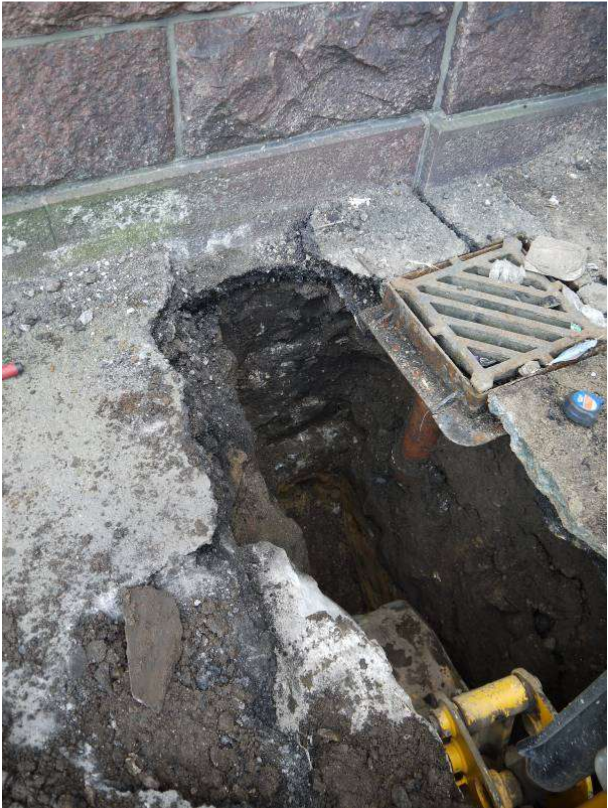
Illustration 23 TP2 excavated to natural and base of wall foundation looking south west
