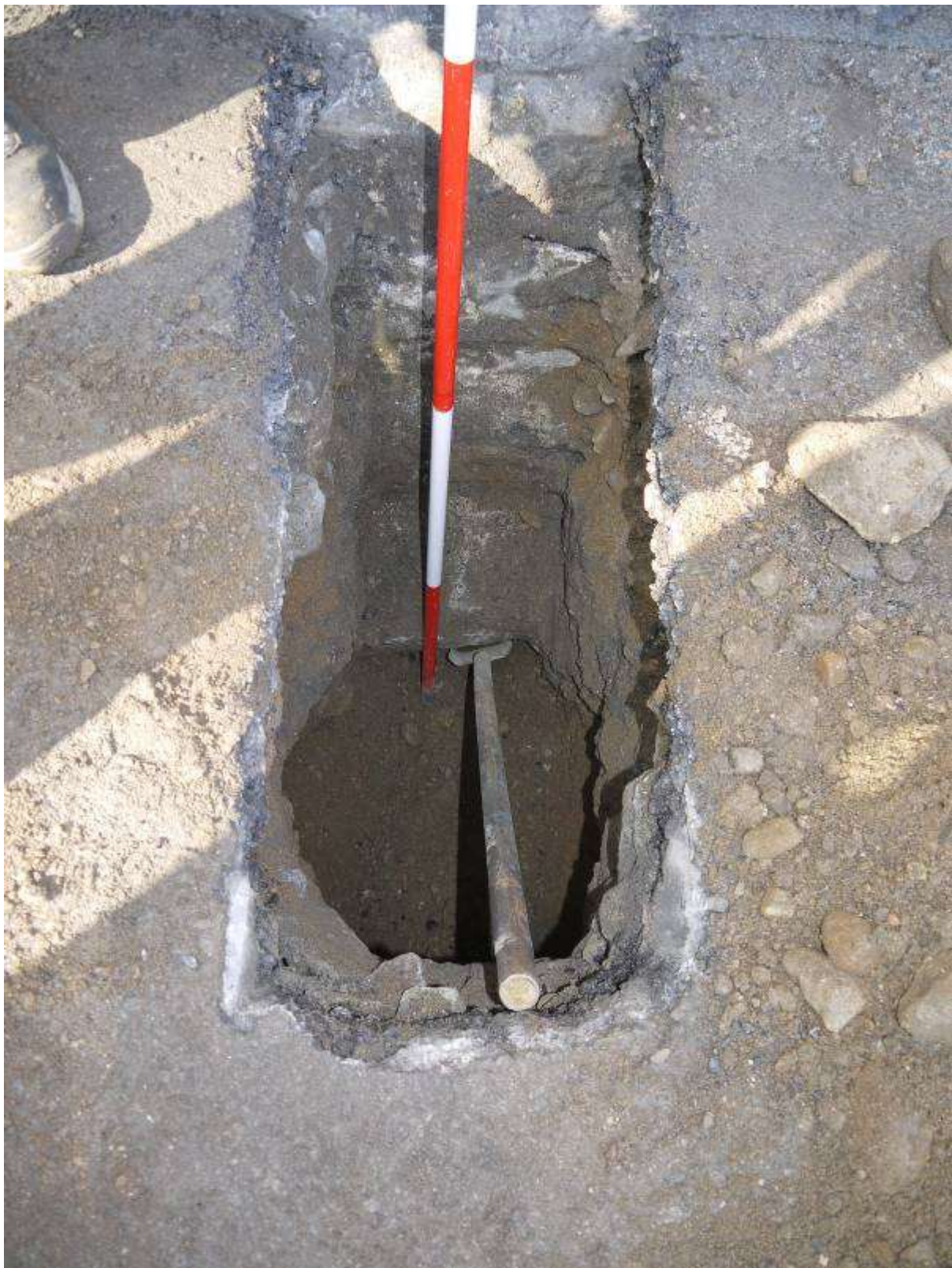
Illustration 31 machine dug trench against east wall of AAG (TPSof3) showing base of foundation
