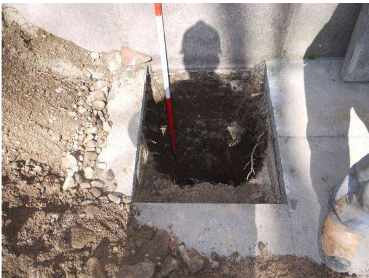
Illustration 20 STP9 excavated to natural and base of wall foundation looking north
