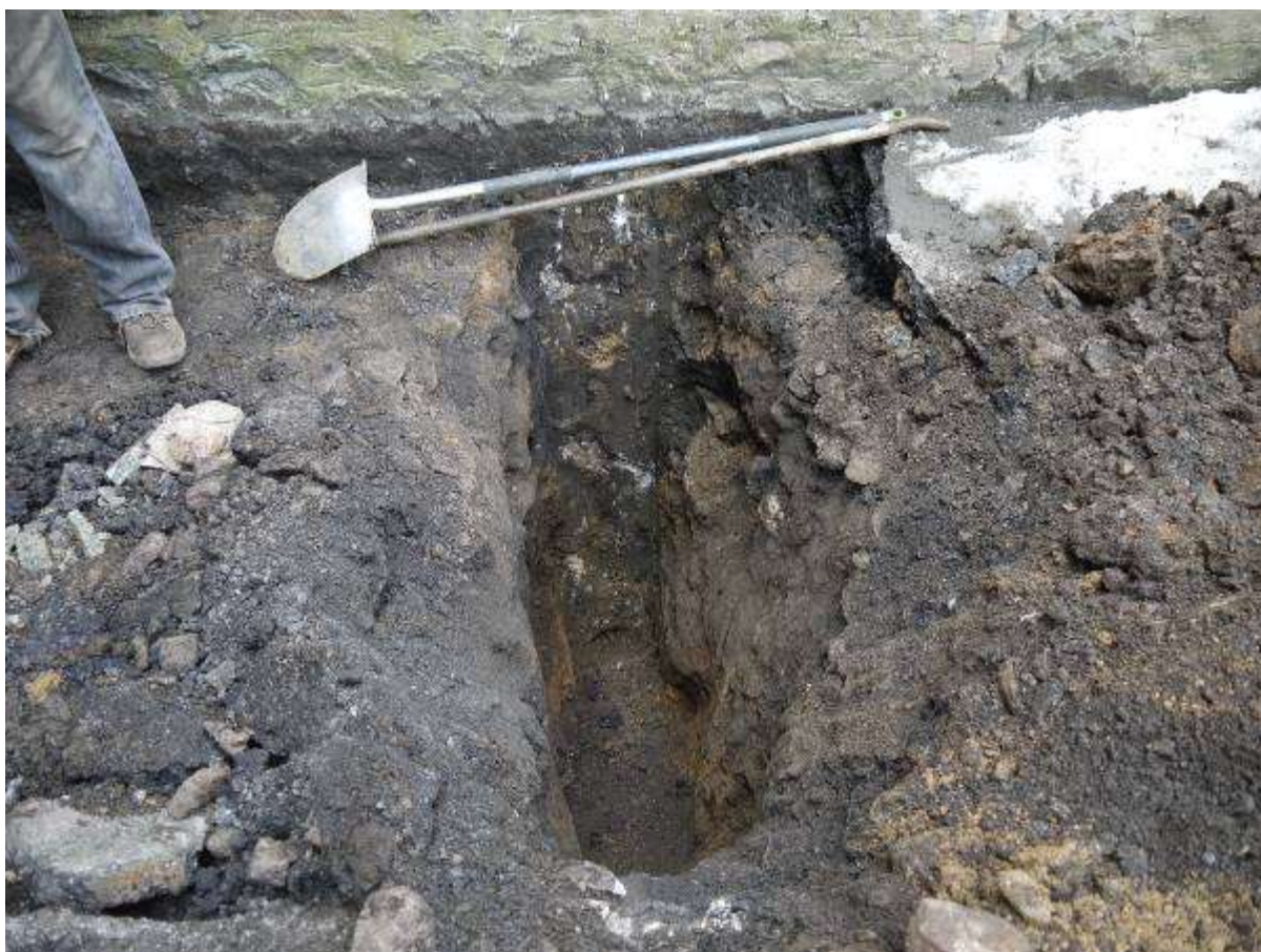
Illustration 33 Machine dug test pit against Robert Gordon's College retaining wall in car park dug to base of wall foundation and natural ground surface looking west
